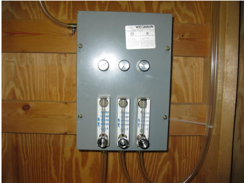
Figure 3.24 Flow Balancing System
