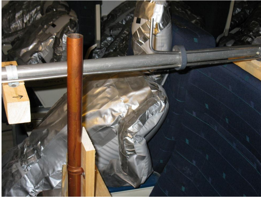
Figure 4.2 Tracer Gas Injection Tube
