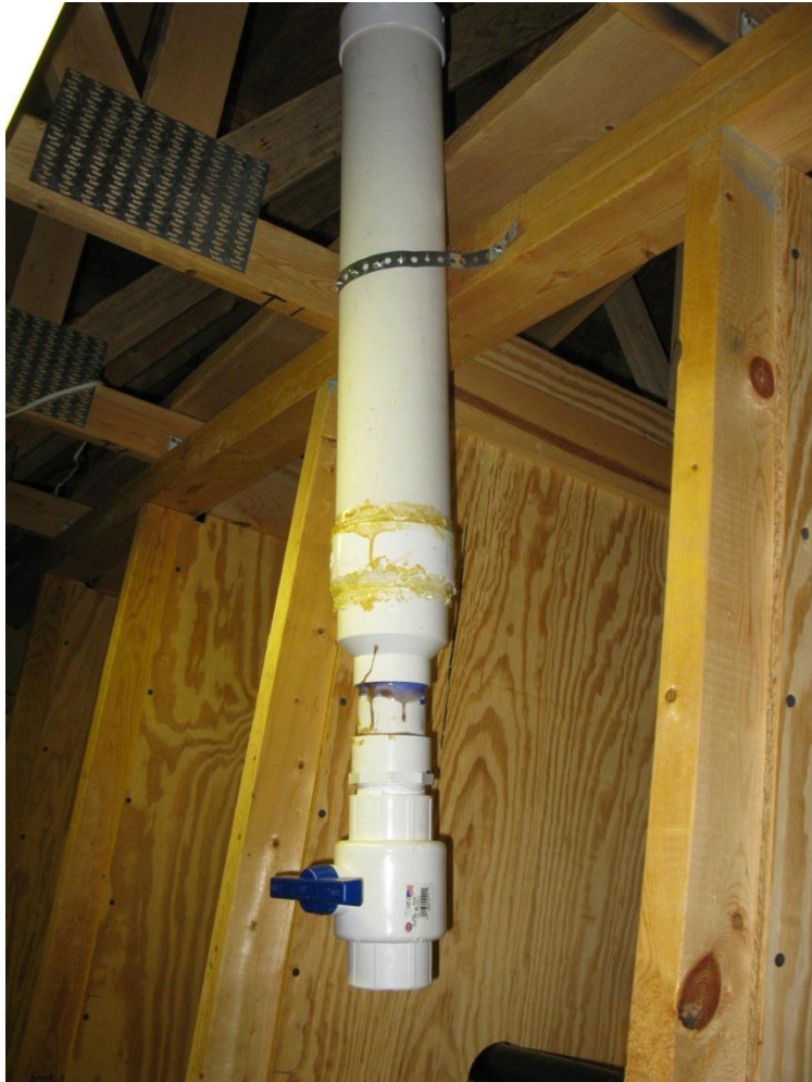
Figure 3.20 Gasper System Pressure Regulator
