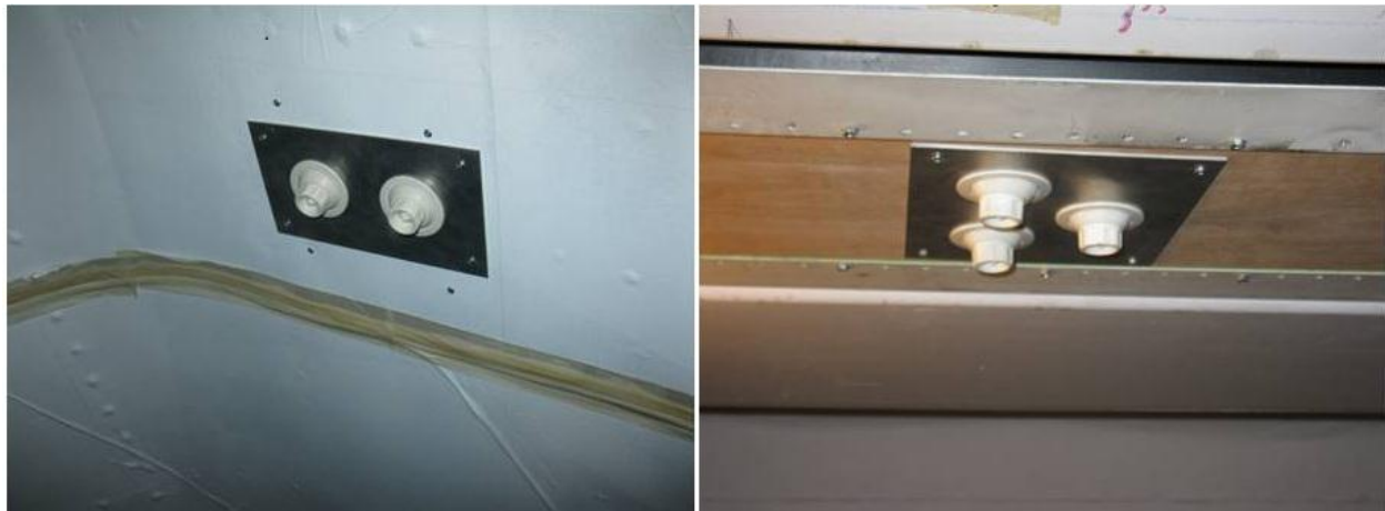
Figure 3.17 Gasper clusters installed in cabin
