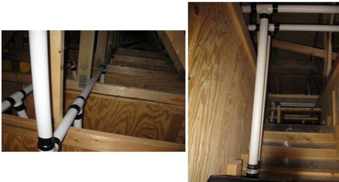
Figure 3.19 Connections from Supply Lines to Gaspers
