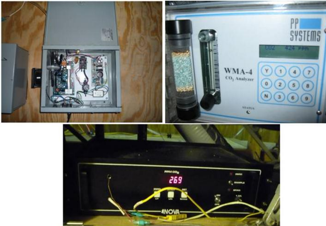
Figure 3.23 CO 2 sensors: Inlet air sensor (top left), NOVA 420 (bottom), WMA-4 (top right)
