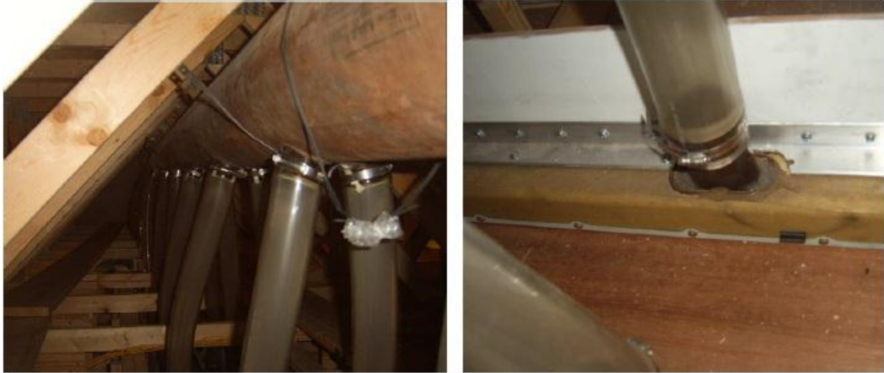
Figure 3.13 Connections of Cabin Ductwork, Flexible Tubing, and Linear Diffusers (Trupka, 2011)
