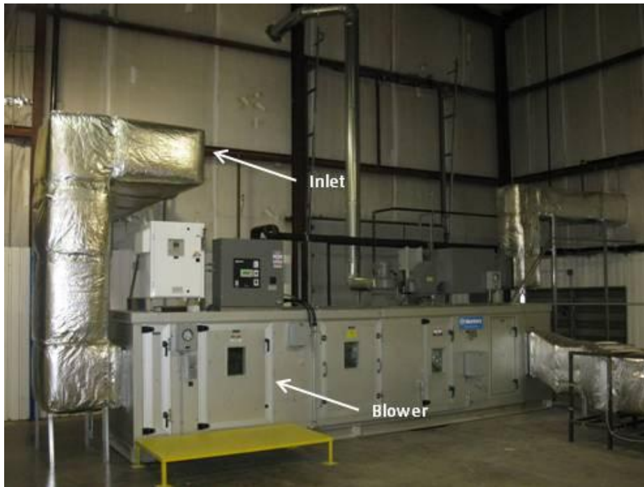
Figure 3.12 Dehumidification System and Current Duct Inlet
