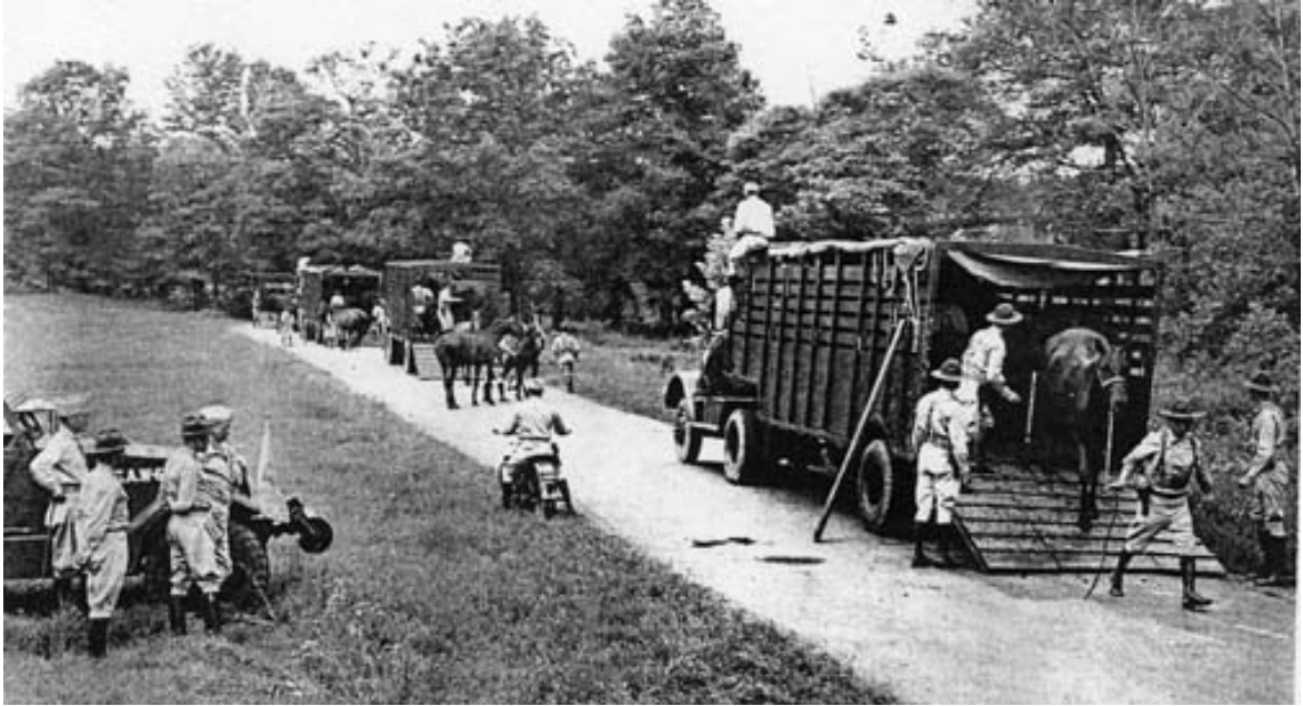
Figure 2-2. Tractor-trailers portee Army cavalry during Louisiana maneuvers in 1940. One tractor-trailer could move eight horses or mules (Cavalry Journal September-October 1940).
