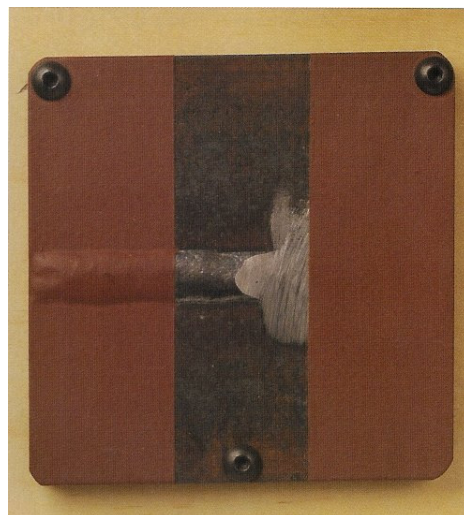
Figure 12: Weld Ground Smooth (Architecturally Exposed Structural Steel, 2003)
