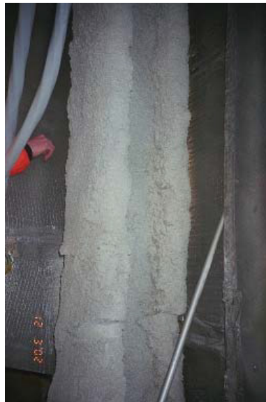
Figure 4: Structural Steel Column Protected with SFRM (Parker, Beitel, & Iwankiw, 2005)
