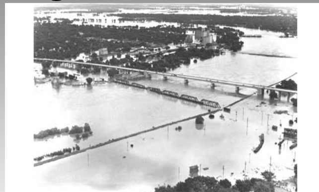
Rock Island railroad bridge and U.S. Hwy. 75 bridge (Topeka Boulevard, center), Melan bridge (Kansas Avenue, upper right), Santa Fe railroad bridge (top right) after washing out. Photo looking northeast (photo courtesy of G.L. Sardou, Topeka, Kansas).
