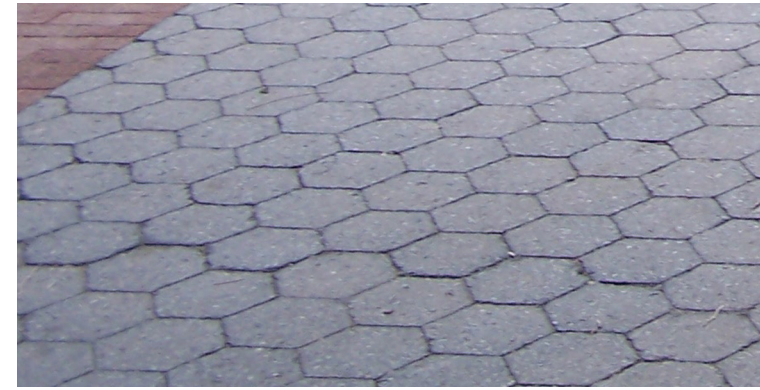
Figure 7.7 Materials - Asphalt Paver
