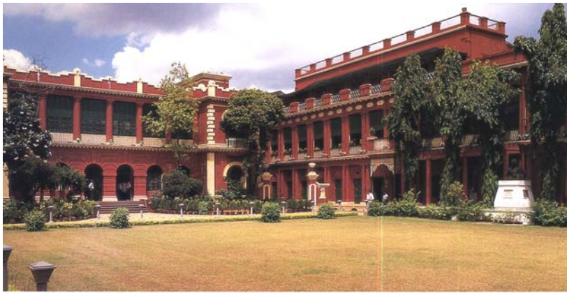
Figure 2.9: Rajbari in Kolkata showing inner courtyard.
