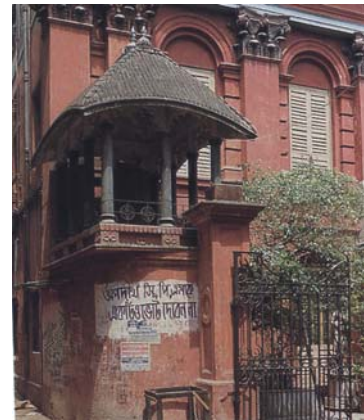
Figure 2.10: Western façade treatment with bangladar roof on top of guard room.
