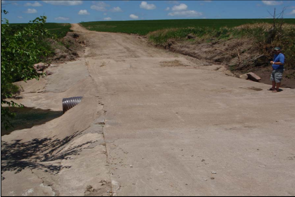
Figure 3.2 Low water crossing at Site 13103. Source; author, July, 2008.
