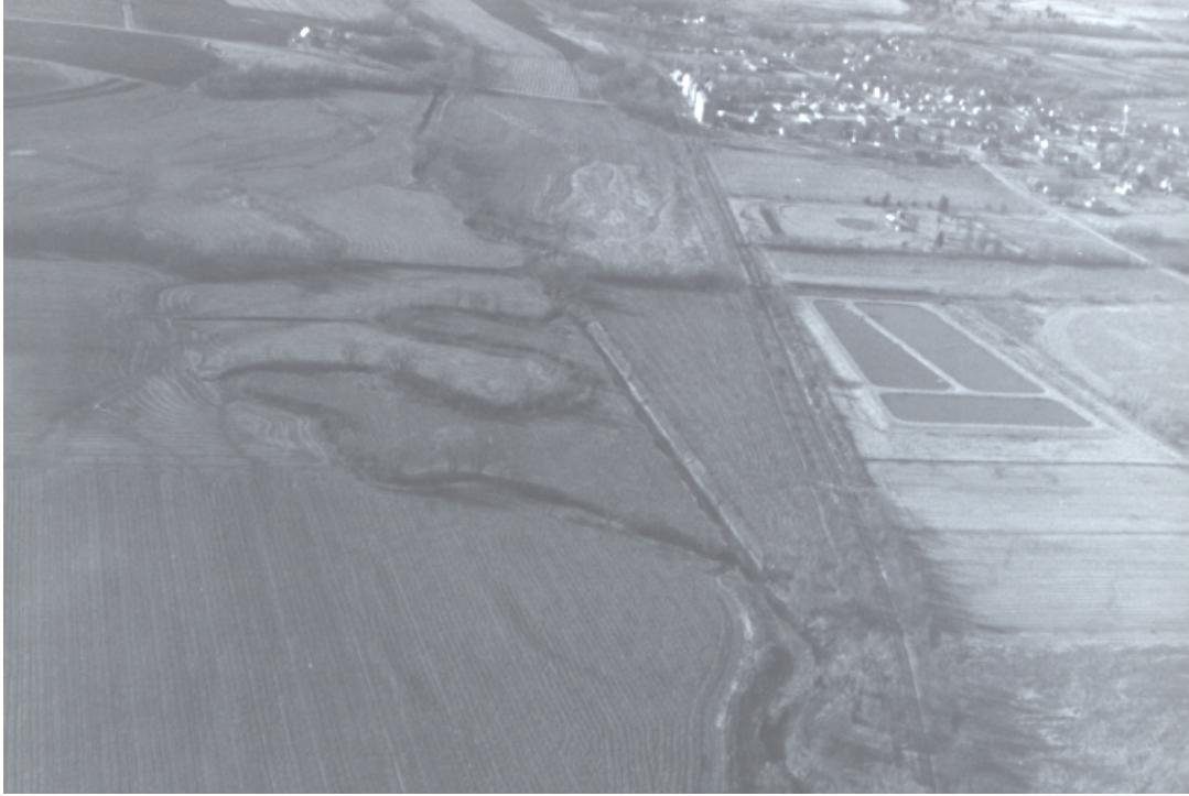
Figure 2.8 Channelization on the Main Branch of the Black Vermillion River near Vermillion, Kansas. Source: Erik Peterson, January, 1987.
