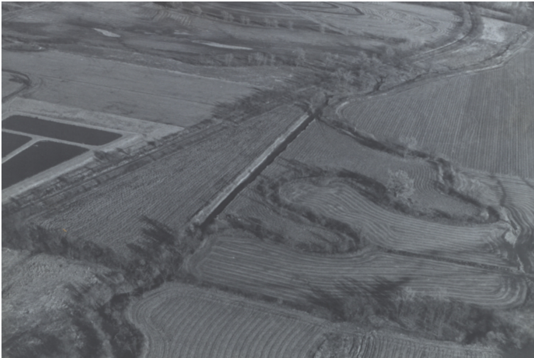
Figure 2.9 Channelization on the Main Branch of the Black Vermillion River near Vermillion, Kansas. Source: Erik Peterson, January, 1987.
