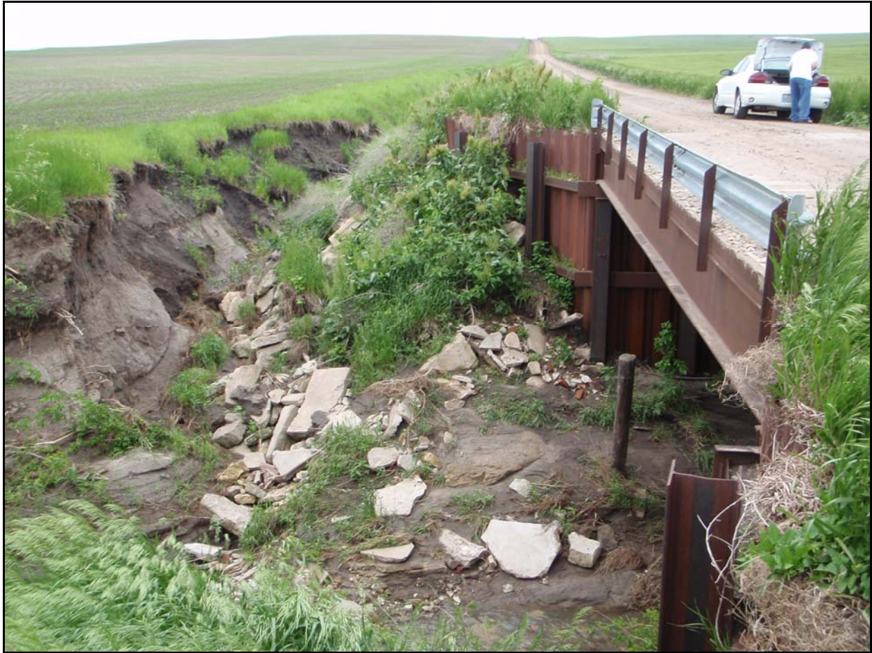
Figure 2.2 Site 13056 looking perpendicular to channel (South). Source: author, May, 2008.
