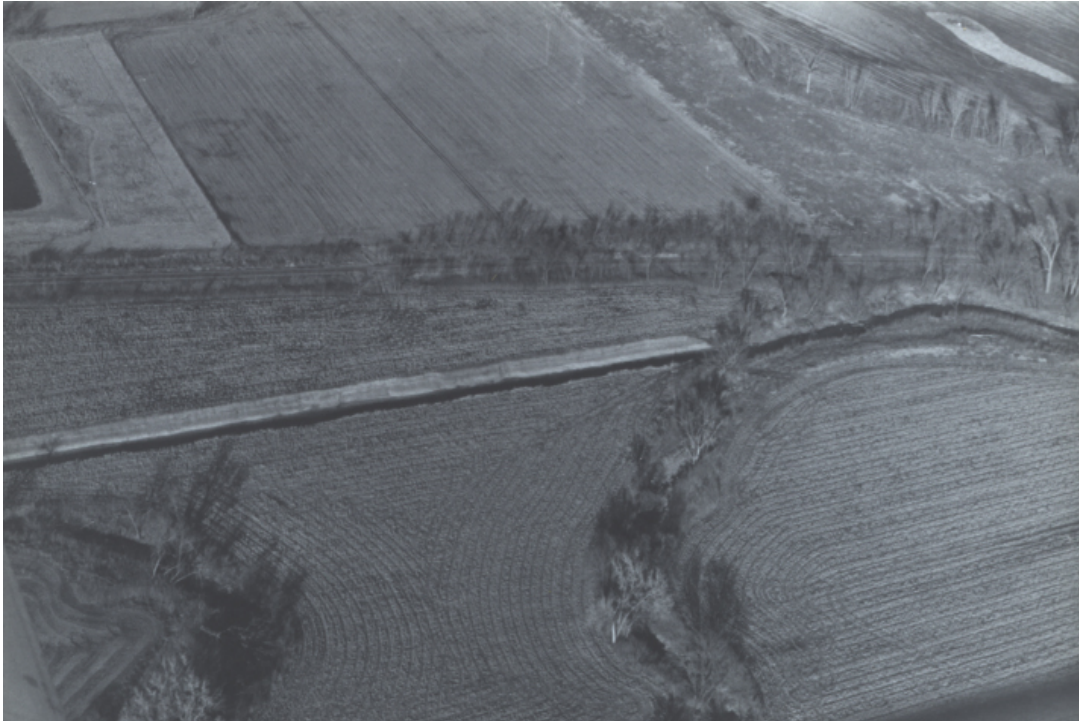
Figure 2.10 Channelization on the Main Branch of the Black Vermillion River near Vermillion, Kansas. Source: Erik Peterson, January, 1987.
