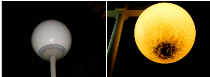
Figure 2.1 Maintenance Issues for the Existing Light Fixtures
