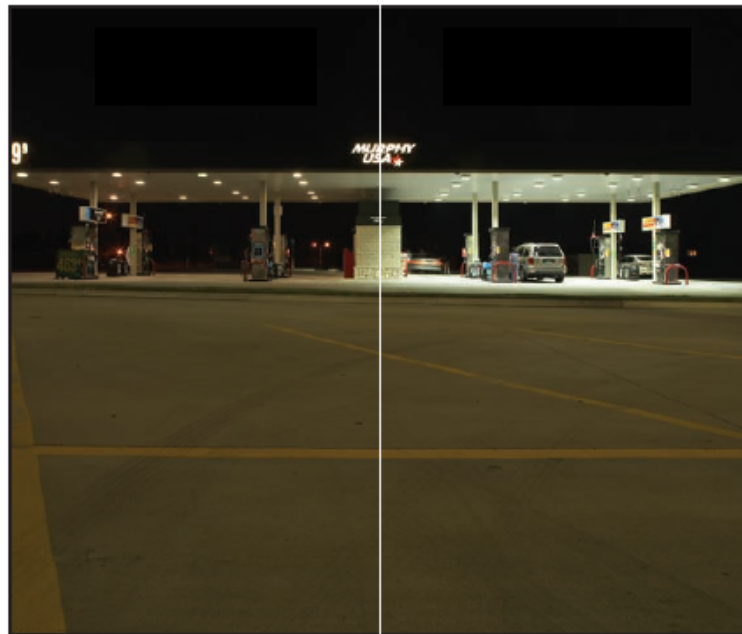
Figure 4.6 Case Study Comparing Metal Halide to LED Lamping
