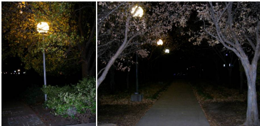
Figure 2.5 Plant Growth Issues for the Existing Light Fixtures
