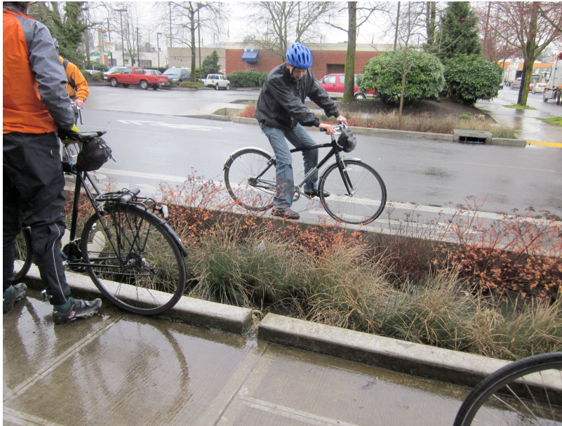
Figure 2.1 Bioswale as Green Infrastructure in Portland, Oregon
