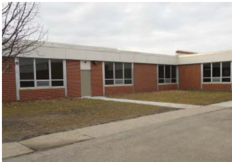
Figure 4.29. Existing Site Conditions. Photo by Author
