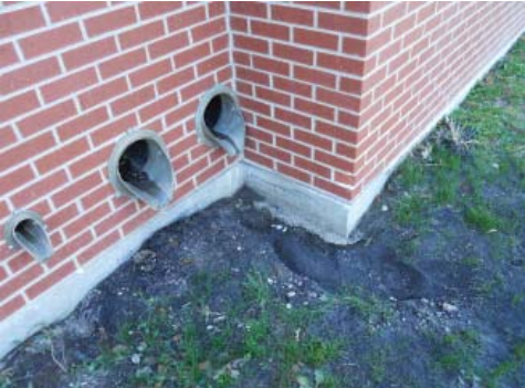
Figure 2.5. Roof drains creating erosion channels. Photo by Author
