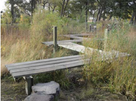
Figure 3.29. Elevated Wetlands Trail. Photo by E. Weatherholt
