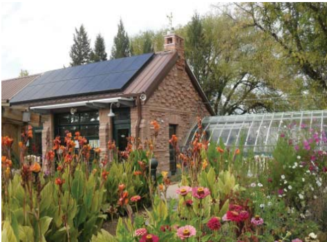
Figure 3.31. Photovoltaics on LEED Certified Children's Center. Photo by E. Weatherholt
