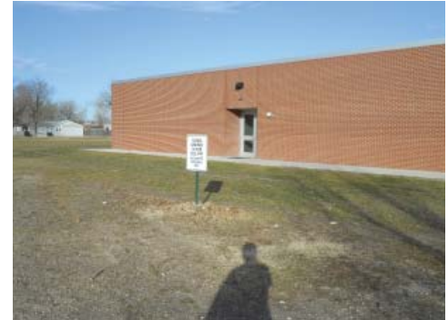
Figure 4.22. Existing Site Conditions. Photo by Author
