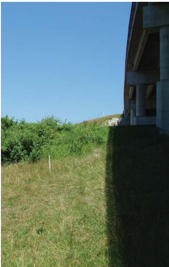
Figure B.01 Pedestrian Bridge Underpass
