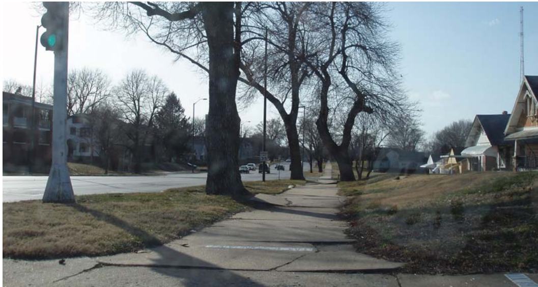
Figure D.09 Poor Prospect Sidewalks
