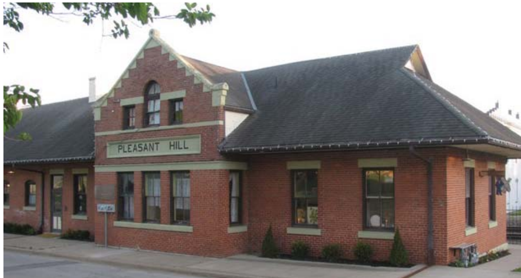
Figure D.05 Pleasant Hill Train Station
