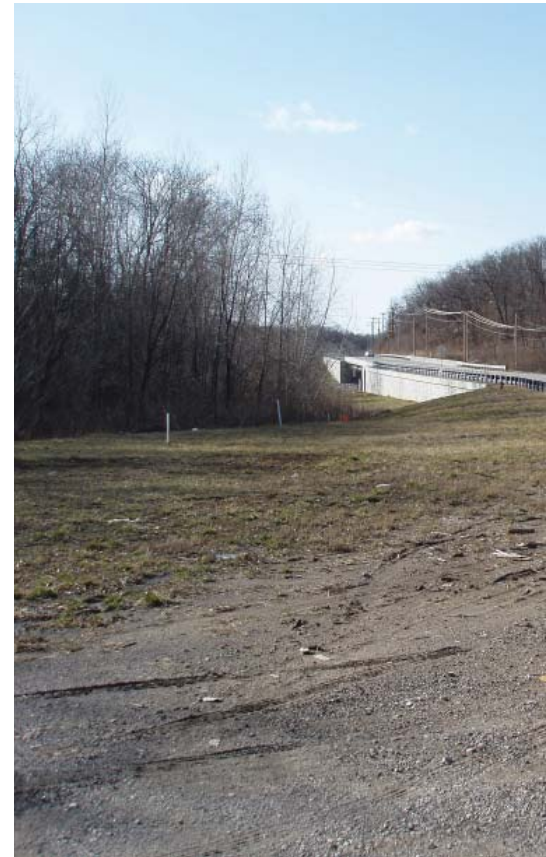
Figure D.11 Raytown Road Bridge
