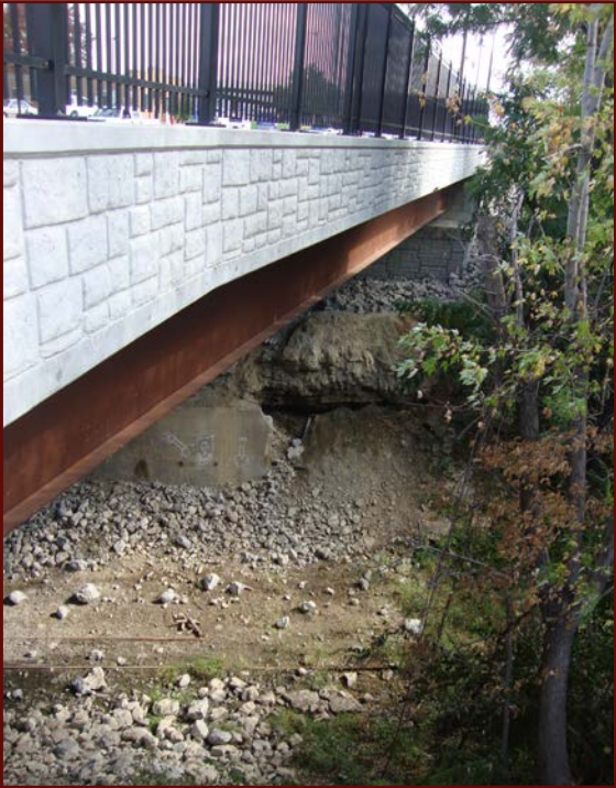
figure 2.03: corridor under raytown bridge.
