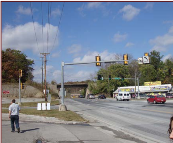
figure 2.04: corridor crossing at knobtown.
