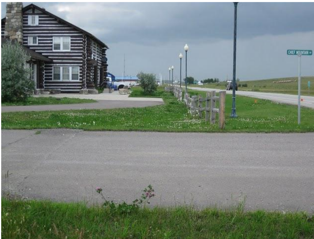
Figure 3.4: The Port of Piegan Border Inspection Station, Montana. The view is from the intersection of U.S. 89 and Chief Mountain Road, facing north. The new, blue-roofed inspection and customs building is visible in the distance. Taking photographs of ongoing vehicle inspections, as the Vales did during the early 1980s, is now strictly forbidden.
