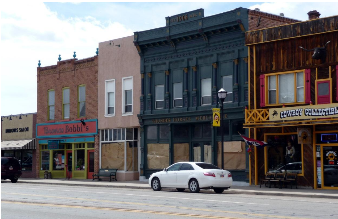
Figure 8.8: Facing Southwest along U.S. 89 through downtown Panguitch, Utah. Date and Time of Rephotography: 2:00pm, Wednesday, March 18, 2009.
