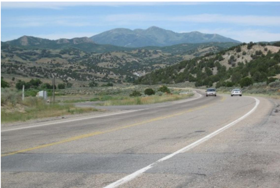
Figure 5.2: This view depicts U.S. 89 immediately to the north of Birdseye, Utah. The view is facing north, toward the former town of Thistle and the Wasatch Mountains. The tallest mountain in the distance is Uinta National Forest's Spanish Fork Peak, at 10,192 feet above sea level. Although the open range sign has disappeared, this is still, by all indications, open rangeland. Date and time of rephotography: 2:00pm, Monday, August 3, 2009.
