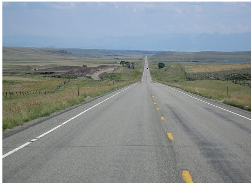
Figure 5.3: U.S. 89 between Wilsall and Ringling, Montana, facing southeast. The Bridger and Bangtail (right), as well as the Absaroka (left) mountain ranges are visible in the distance, though are obscured by haze in the 2009 image. Cottonwood Reservoir is also visible in both images at the center right. Date and Time of Rephotography: 3:30pm, Sunday, August 12, 2009.
