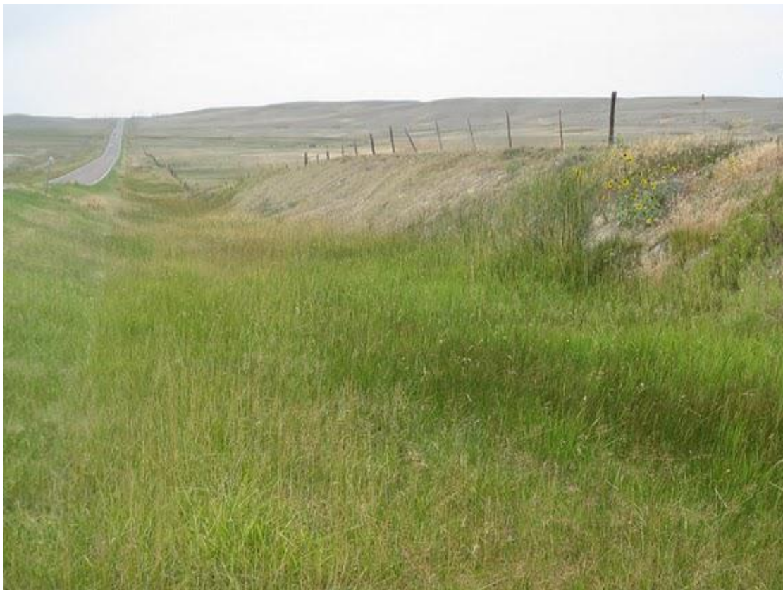
Figure 5.5: U.S. 89, approximately thirty miles northwest of Great Falls, Montana. The view is facing northwest, and the structures visible along the road in the distance are power lines. Date and Time of Rephotography: 2:00pm, Sunday, August 16, 2009.
