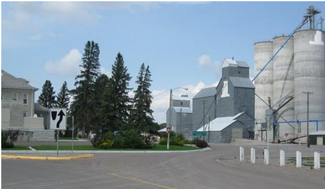
Figure 8.3: Choteau, Montana, at the roundabout that serves as the intersection of U.S. Highways 89 and 287. The view is facing north, and the building on the far left is the Teton County Courthouse.
