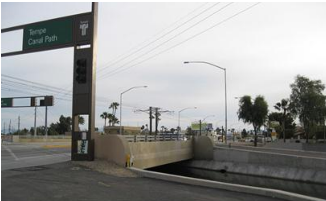
Figure 9.10: The view eastward into Mesa, Arizona from the Tempe bank of the Tempe Canal. The road adjacent to the photographer’s position is Apache Boulevard East (Tempe) and West Main Street (Mesa). Though the City of Mesa’s prominent welcome sign viewed in the Vales’ photograph no longer exists, a “Welcome to Tempe” marker stands immediately to the left (north) of the area depicted here.
