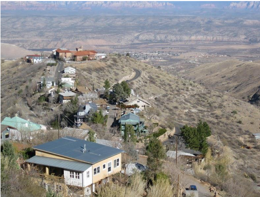
Figure 8.10: A view of Jerome, as seen from a now-blocked off scenic pull off along Arizona State Route 89A to the southwest of the city. The view is facing northeast, into the Verde River Valley and to the cliffs of the Mogollon Rim beyond. Date and Time of Rephotography: 2:20pm, Saturday, January 9, 2010.
