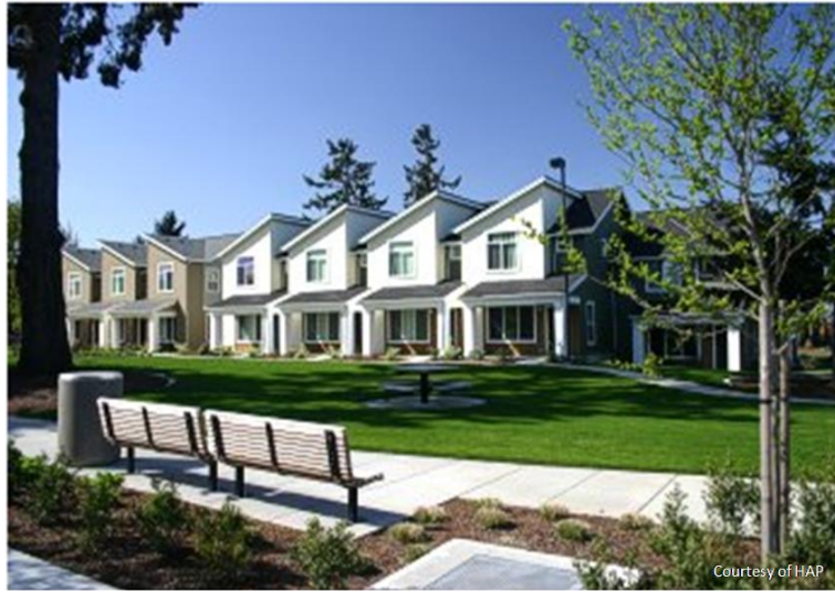
Figure 7.20 Apartment Homes located along North Trenton Street
