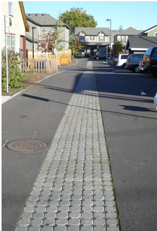
Figure 6.13 Permeable Pavers Located in Alleys
