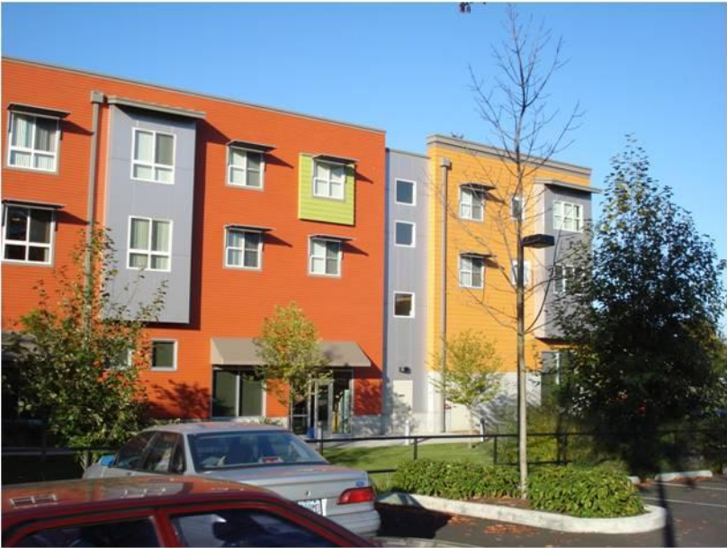
Figure 7.26 Backside (south side) Trenton Terrace
