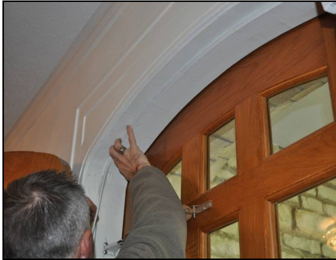
Figure 4.14 Installing New Weather Stripping
