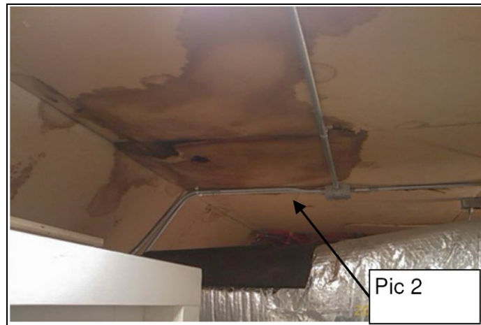
Figure 4.8 Third Floor Mechanical Room Air Leakage
