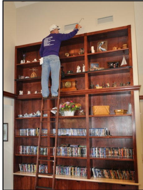
Figure 4.18 Sealing the Crack Above Bookshelf
