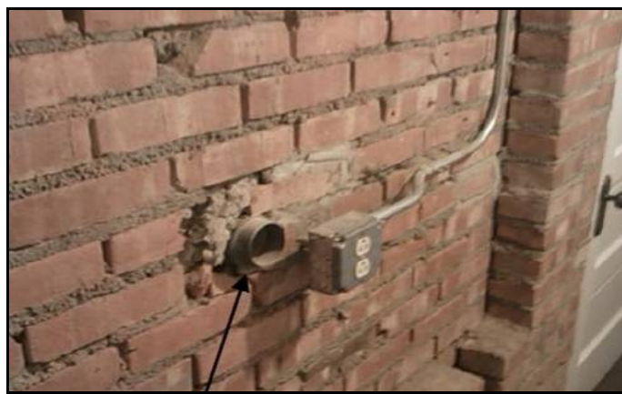
Figure 4.19 Open Conduit in Basement
