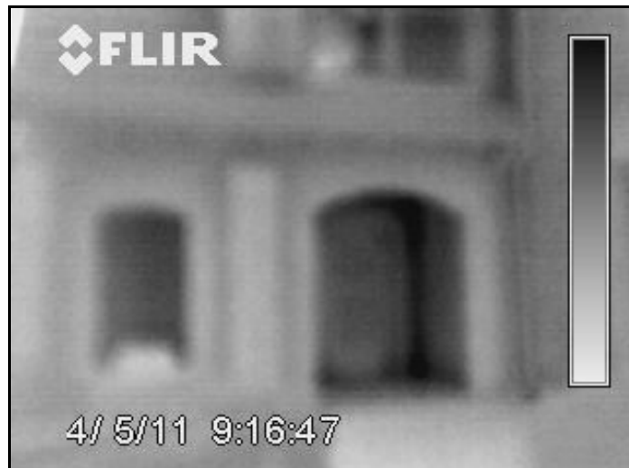
Figure 4.13 Front Door Thermal Image with Old Weather Stripping
