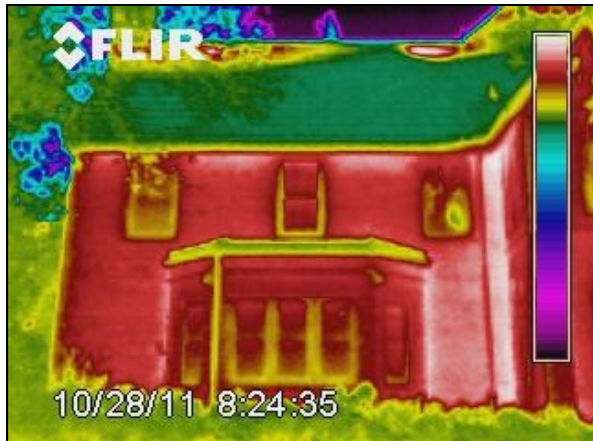
Figure 4.25 President's Residence Thermal Image After Insulation
