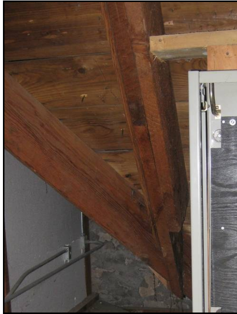
Figure 4.21 Un-Insulated Ceiling
