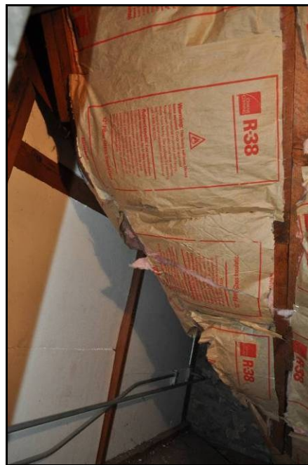
Figure 4.22 Insulated Ceiling
