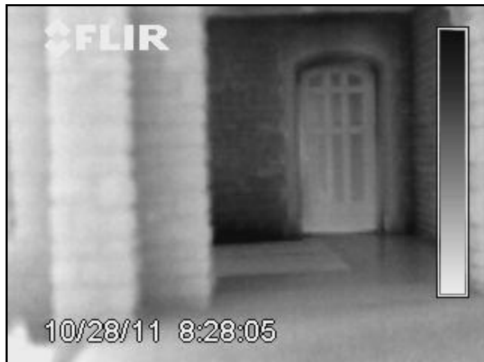
Figure 4.15 Front Door Thermal Image with New Weather Stripping
