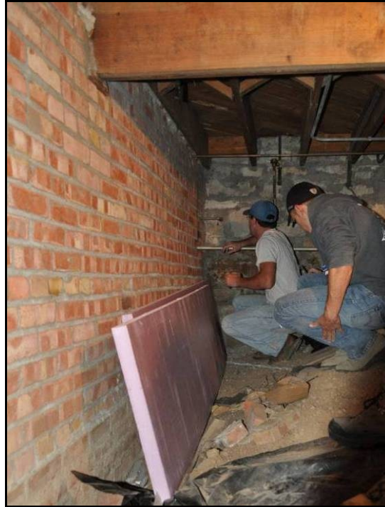
Figure 4.27 Un-Insulated Crawl Space
