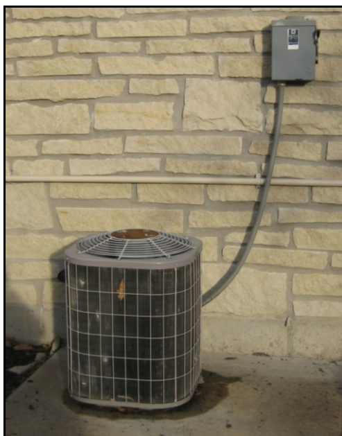
Figure 2.4 Outdoor Condensing Unit
