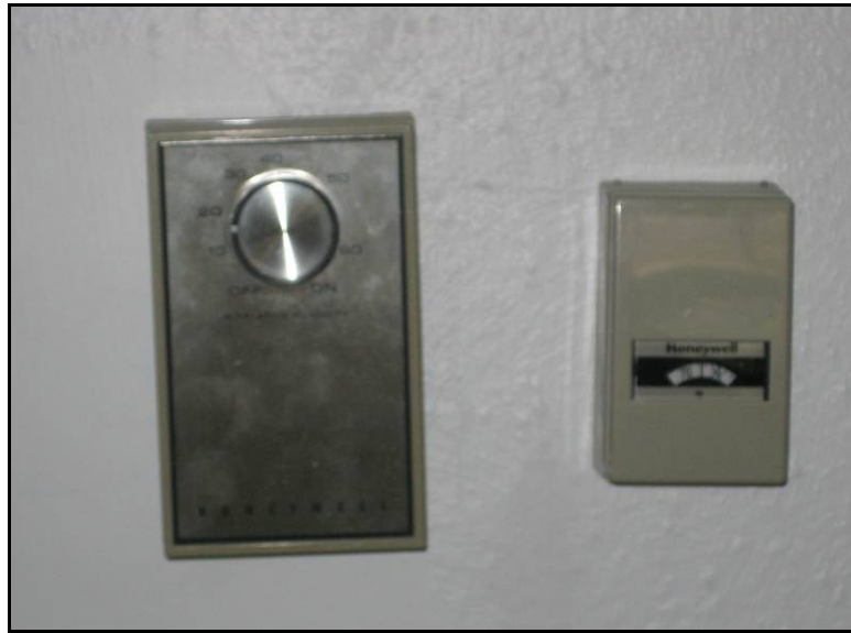
Figure 4.1 Upper Landing Existing Thermostats
