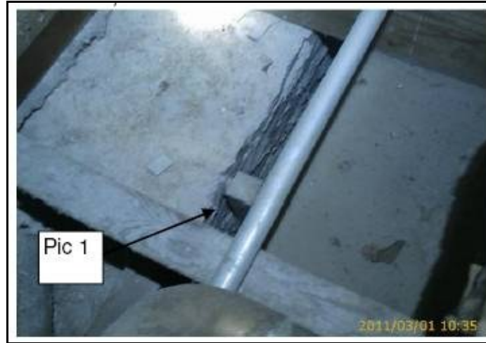
Figure 4.7 Exterior Wall Air Leakage (Energy Audit)
