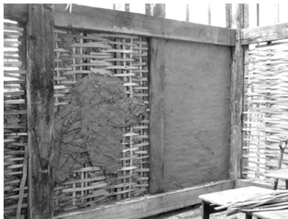
**FIG. 6 WATTLE AND DAUB CONSTRUCTION**
