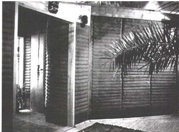
**FIG. 8 STRANGLEHM TYPE OF CONSTRUCTION**
