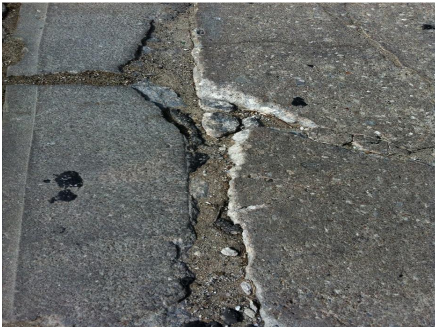
Figure 2-2: Joint rot in which poor quality aggregates, can be seen popping out of the concrete pavement at the joints.
