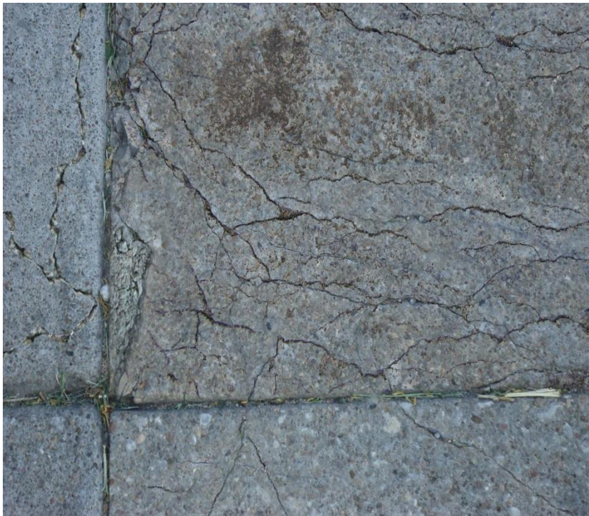
Figure 2-3: D-cracks (low intensity) observed near joint on College Avenue.
