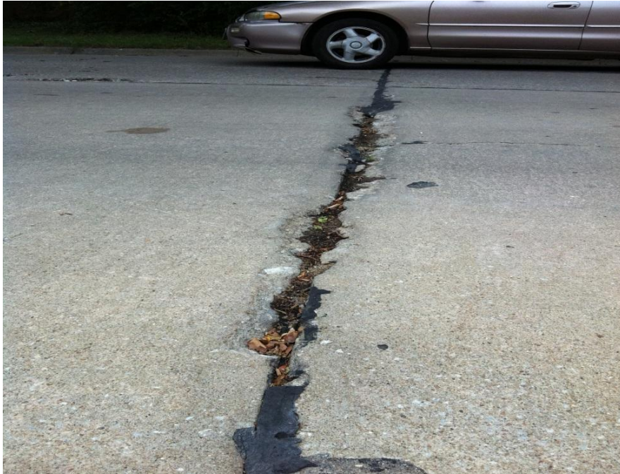
Figure 2-1: Joint rot observed in concrete pavement near Claflin-Denison Intersection.
