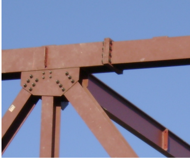
Figure 6.8: Top chord splice connection
