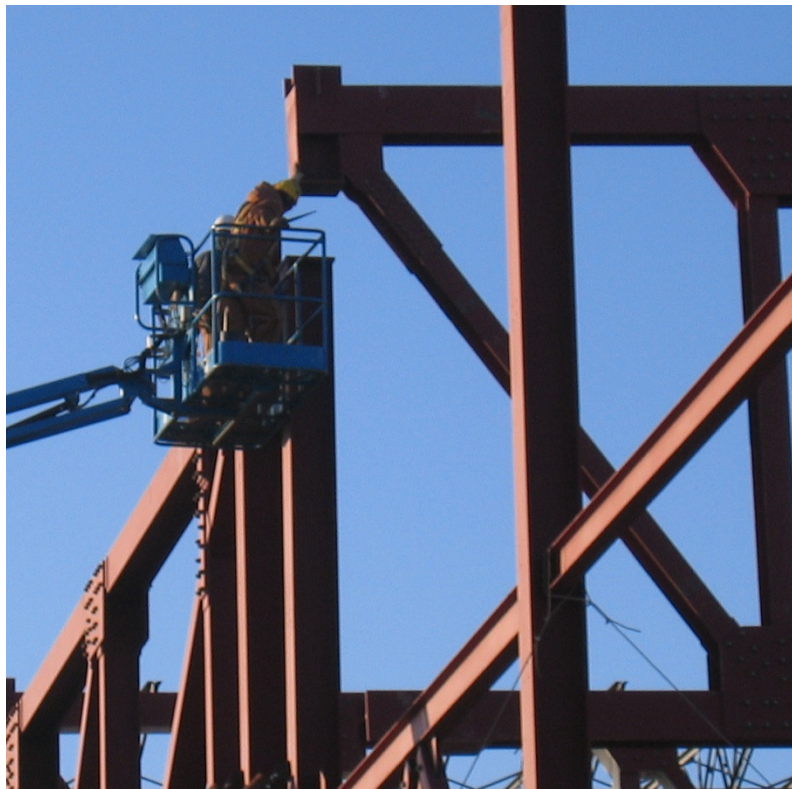
Figure 6.1: Top chord bearing truss being set on column.
