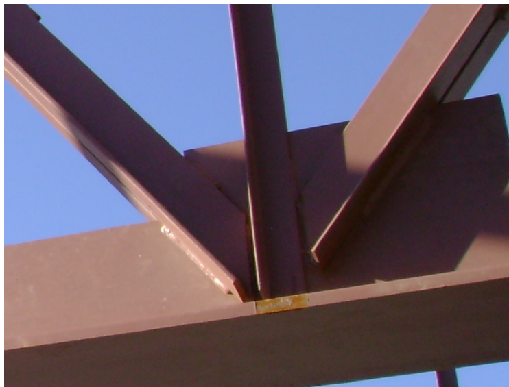
Figure 6.5: Welded chord to web connections.
