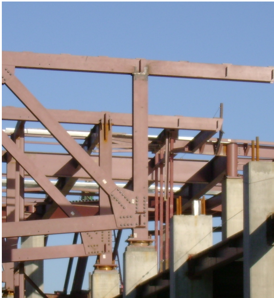
Figure 6.2: Bottom chord bearing truss
