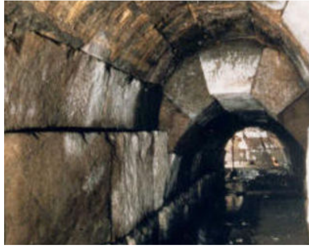
Figure A.2: Stone vault of storm sewer in Munich, Germany
