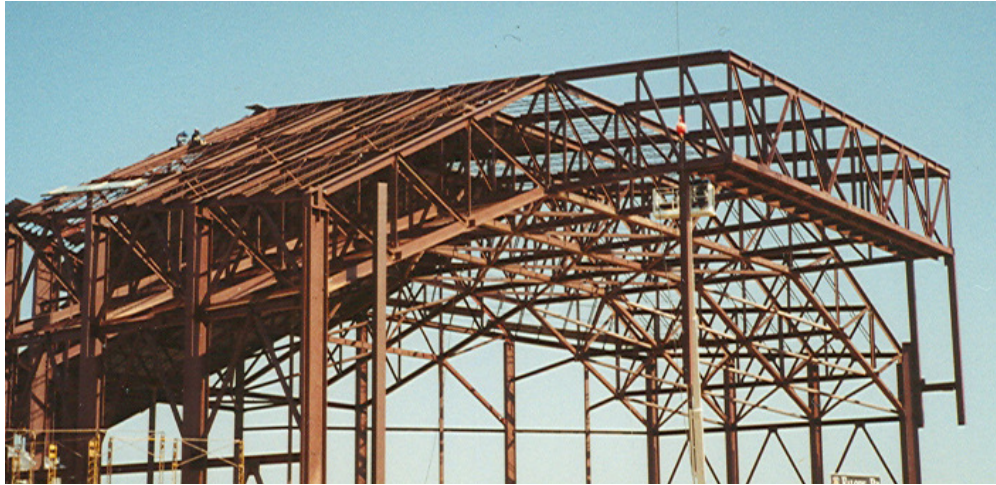
Figure A.8: Steel framework and trusses for an aircraft hanger under construction
