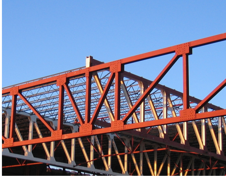
Figure 6.4: Top chord bearing truss.
