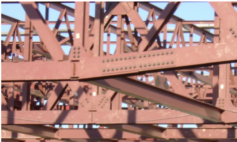
Figure 6.9: Bottom chord splice
