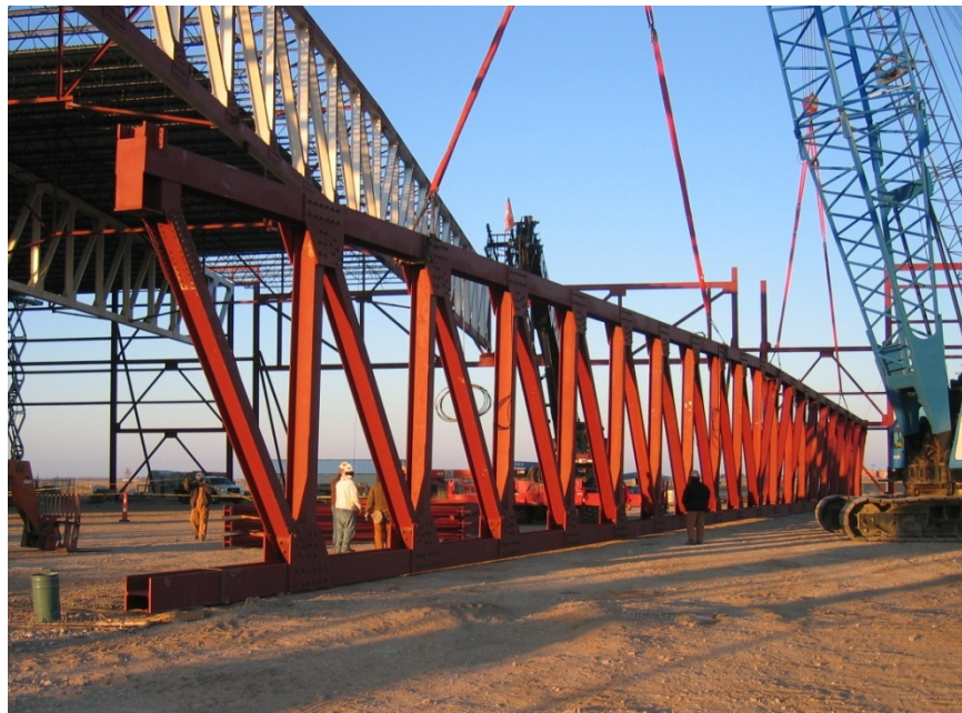
Figure 8.1: Bolted truss assembled at job site.
