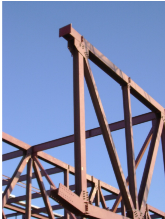
Figure 6.7: Truss before splicing
