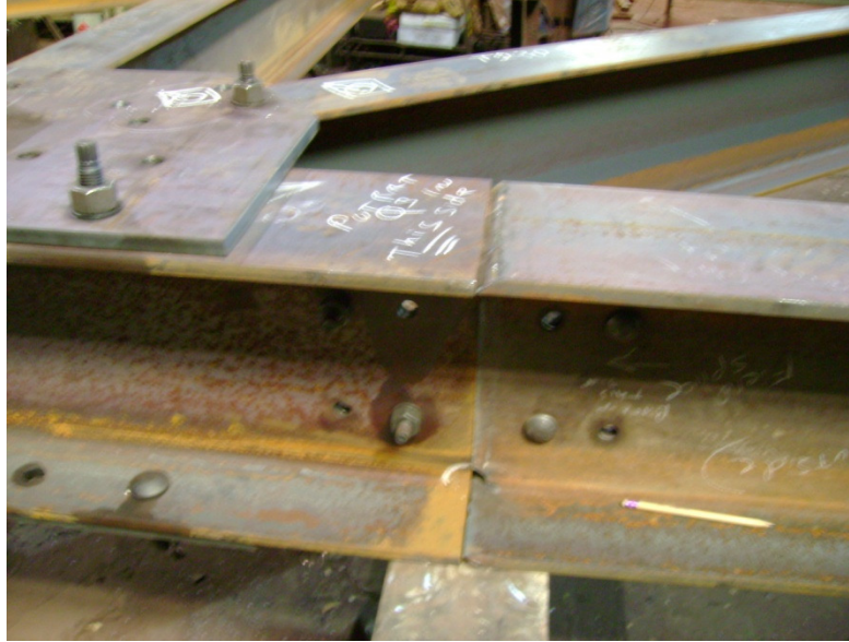
Figure 6.6: Member size change at splice location
