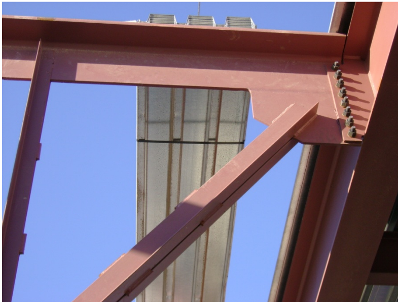
Figure 6.3: Shear connected truss
