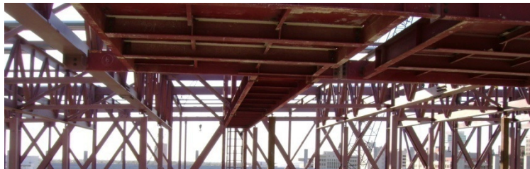
Figure 7.1: Main truss being braced by smaller trusses.
