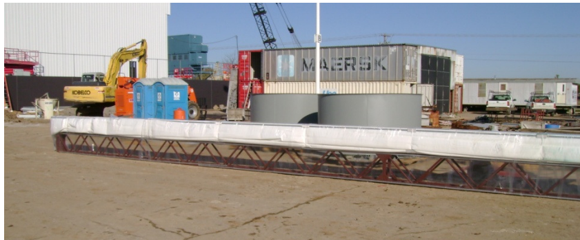
Figure 8.2: Truss recently unloaded off a trailer.
