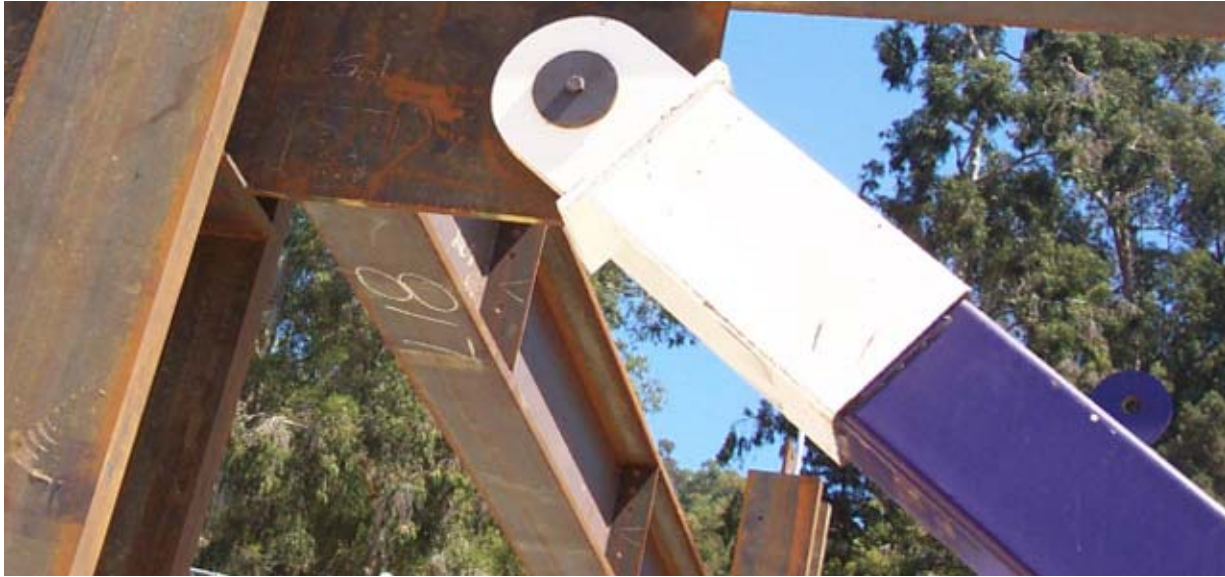
Figure 3-4. True pinned connection [courtesy of Star Seismic, LLC. < http://www.starseismic.net/powercat.php >].
