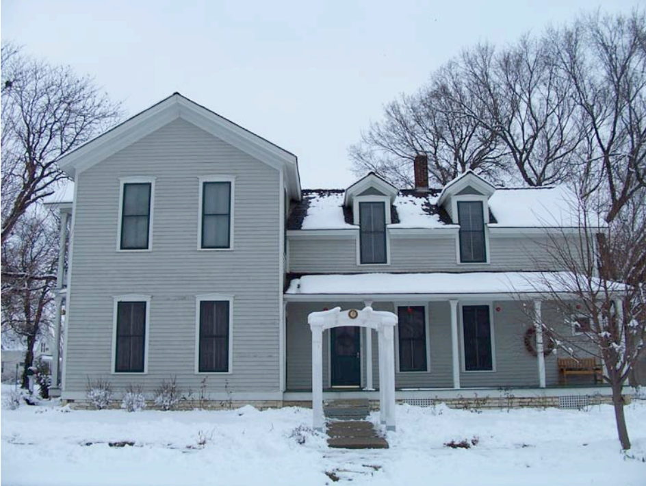
Figure 2-3: Front house West facade
