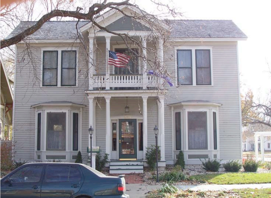
Figure 2-4: Front house North facade
