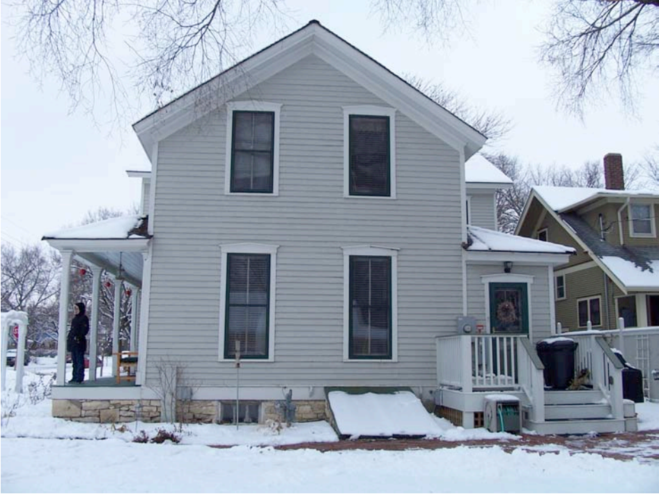
Figure 2-6: Front house South facade.
