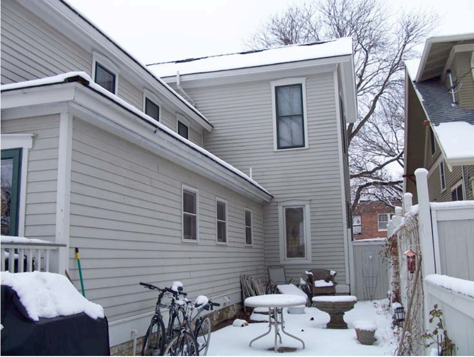
Figure 2-5: Front house East facade.
