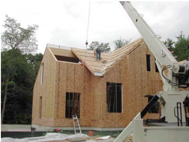
Figure 3-43: Sample SIP construction.
