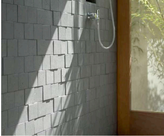
Figure 3-47: Sample concrete bathroom tiles.
