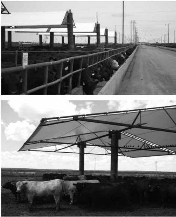
Figure 1. Shade was provided using 13 ounce polyethylene product (Cattle Cabana, Accu-Steel Inc., Templeton, IA) and structures were positioned along both fence lines so that shade was shared between adjacent pens. Water tanks (Johnson Concrete Products, Hastings, NE) were positioned within the fence line so that cattle had access to water while under shade.
