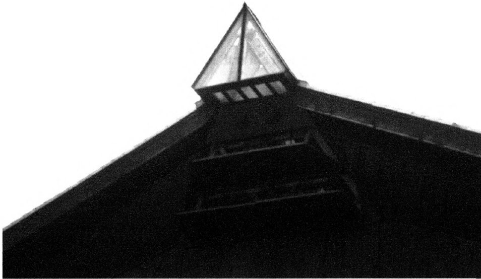
Fig 2.12: The triangular openings help natural ventilation in the main exhibition and the exhibition halls.
