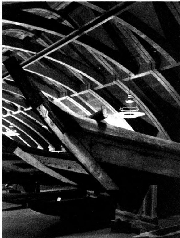
Fig 2.28: The interior space of the repository of ships.
