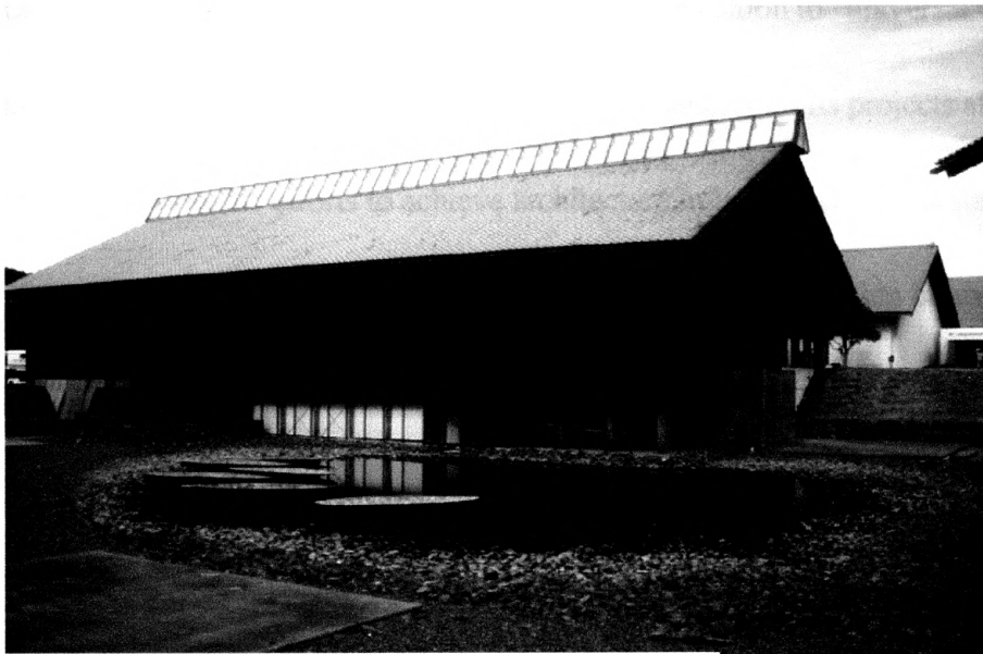
Fig 1.8: The exterior of the main exhibition hall
