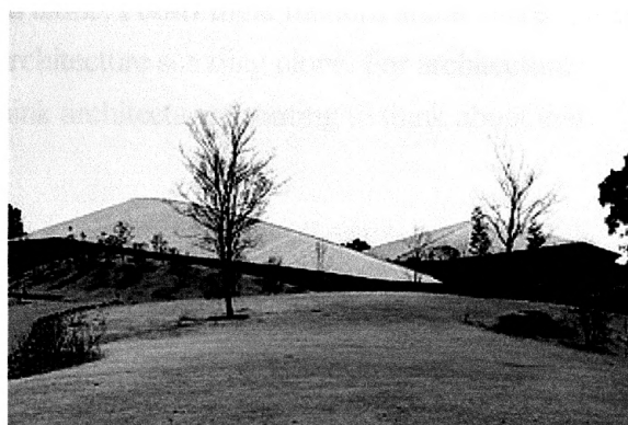
Fig 3.4: The roof of the exhibition hall from the lower level.
