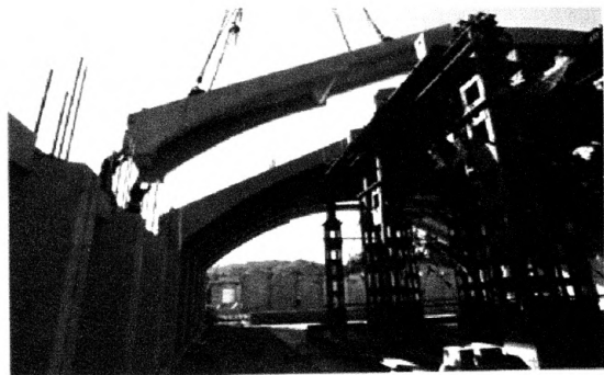
Fig 2.10: The site assembly of pre-cast concrete frames.
