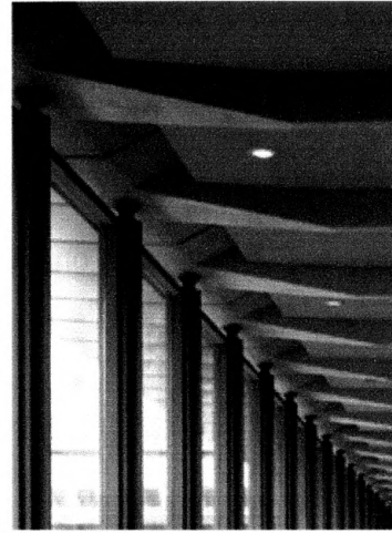
Fig 5.13: The heat-press-shaped steel member has a roll to support roof structure as well as a reinforcing wooden such.
