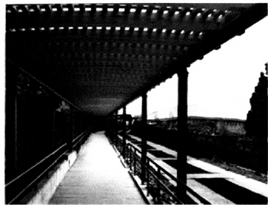
Fig 2.43: The wooden pergola to connect between the two buildings.
