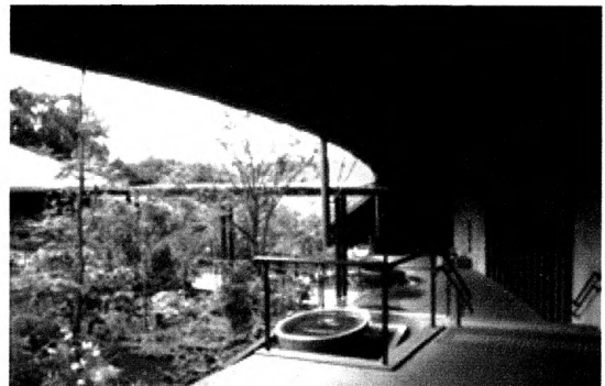
Fig 2.47: The building form follows the topography.
