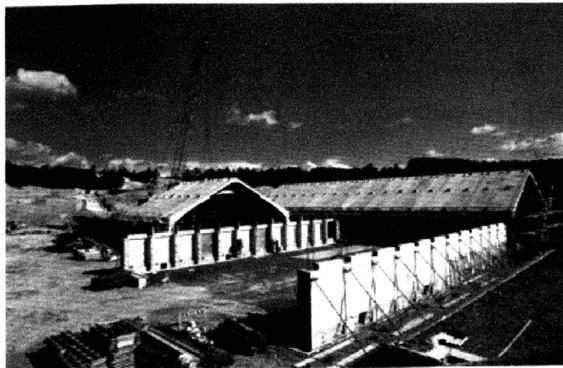
Fig 2.9: The construction process of the repository.
