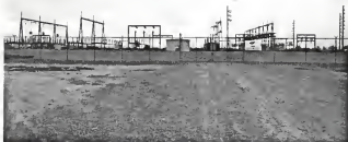
FIGURE IV TYPICAL 230/69 KV RECEIVING STATION
