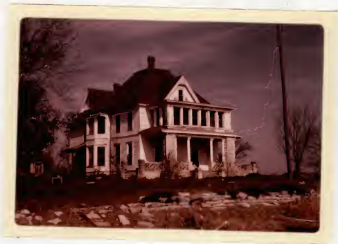
Abandoned Homes near Westmoreland
