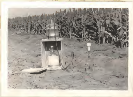
Fig. 2. Method and equipment used to fill atmometers.
