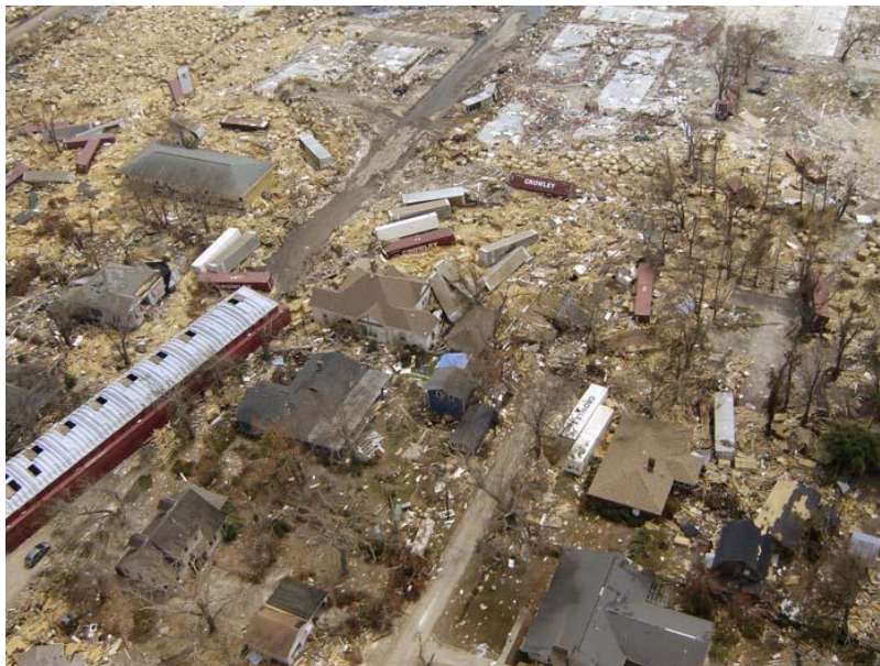
Figure 3.5 Gulfport, Mississippi Houses Moved Out to Sea
