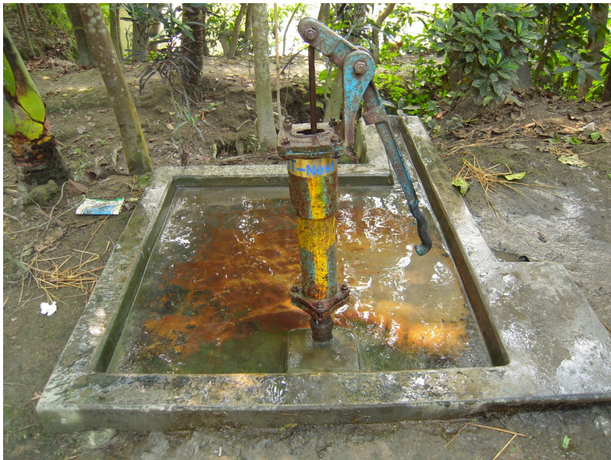
Figure 4.2 Example of a handpumped well which was used for drawing water from aquifers.
