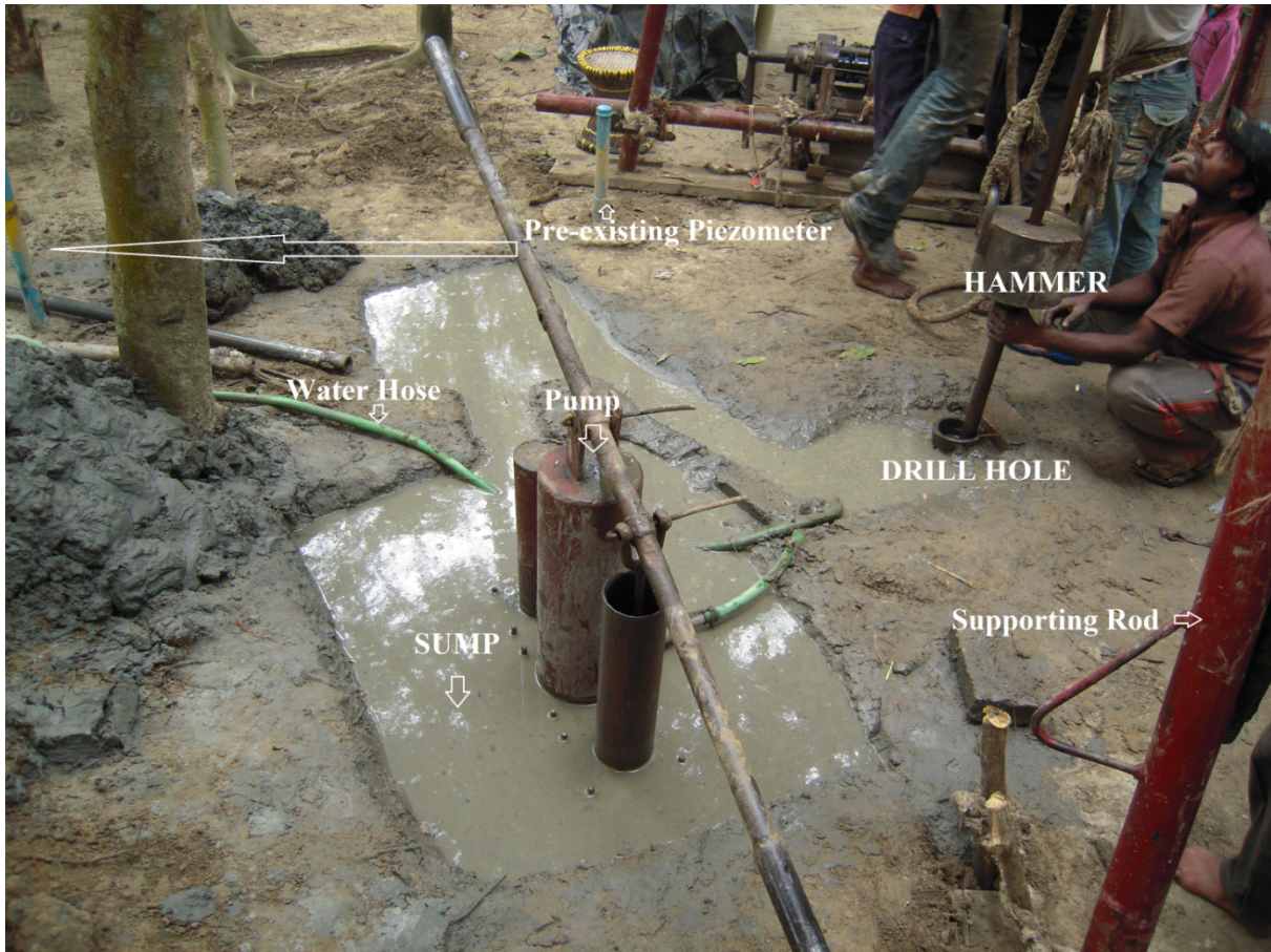
Figure 4.5 Rotary wash boring in North Matlab site (Nest 7)
