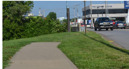
Figure 2-15 | Image of Typical Dead End Sidewalk (Patterson, 2014)
