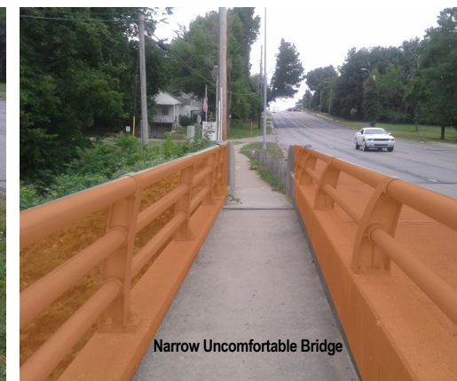
Figure 4-56 | Narrow Confining Bridge (Patterson, 2014)
