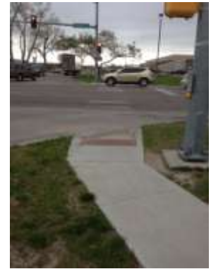
Figure 9. Crossing at Trooper Drive.
