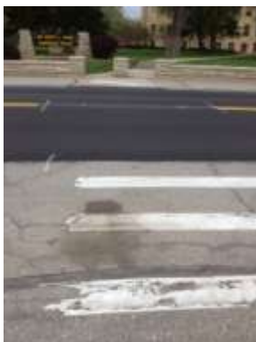
Figure 10. Crossing at Huebner Road.
