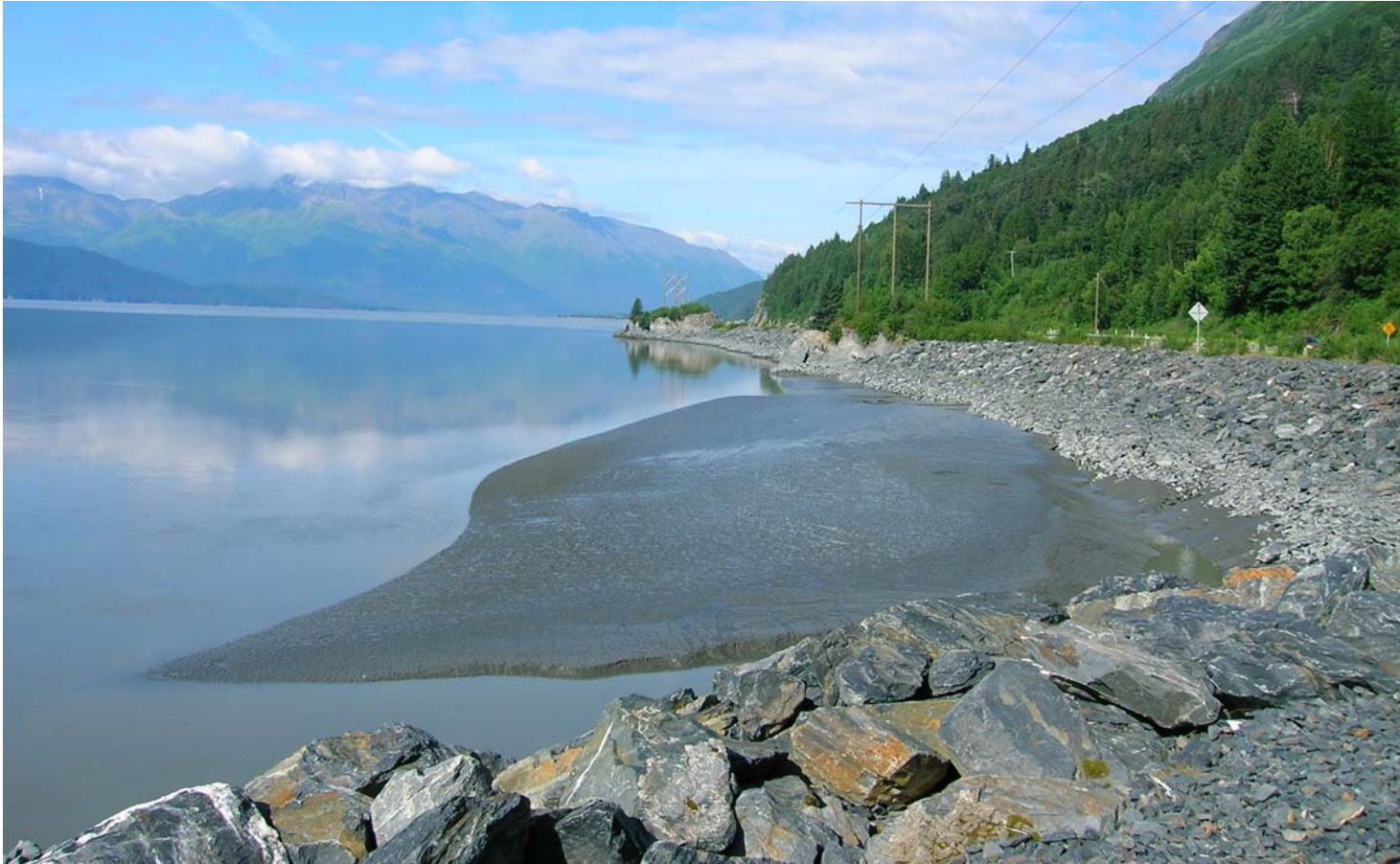
Figure 5-22: TBO4 on July 29, 2007, dewatering from high tide #0.
