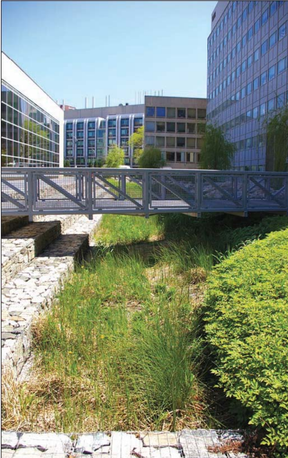
Figure 2.7 Steel bridge over the “river”—MIT’s Stata Center (Source: Echols & Pennypacker, 2006).
