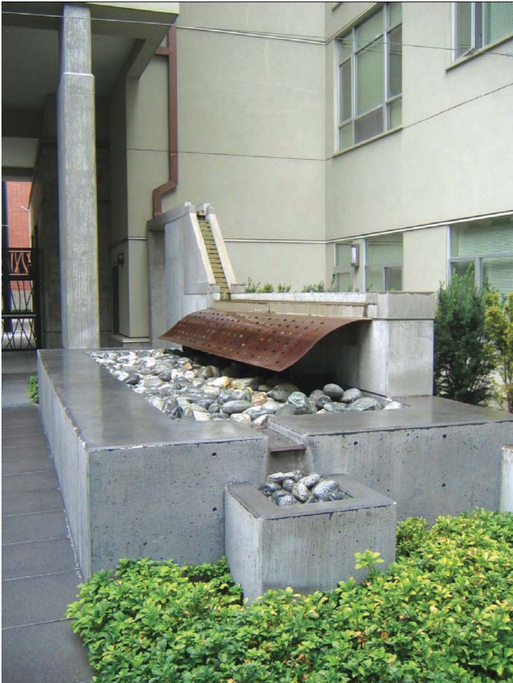
Figure 2.3 Rainwater is conveyed from building roofs to river rock basins through downspouts and runnels—10 th @Hoyt Courtyard
