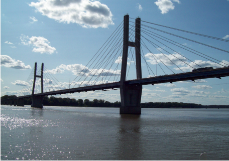
Figure 1-1. Bayview Bridge, Source: Author
