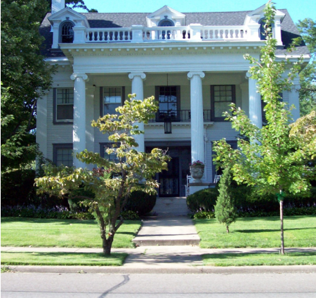
Figure 3-14. Example of historic Quincy architecture; Source: Author
