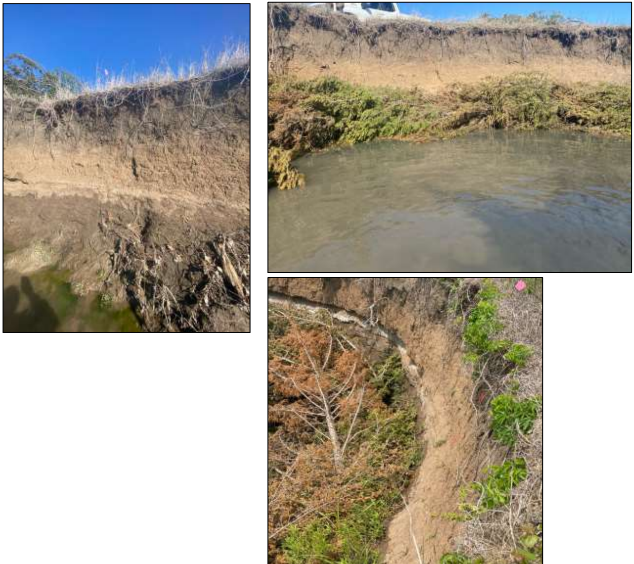
Figure 3.13 Picture of R4 site before and after the installment of the revetment.
