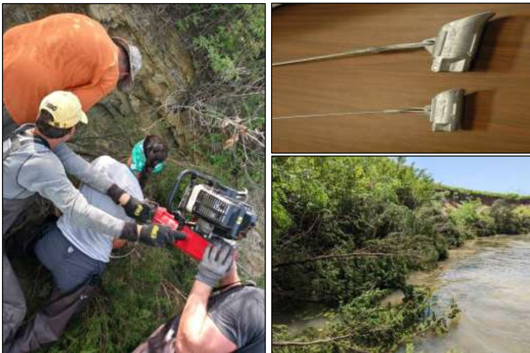
Figure 2.2 Visual example of the installation of R3 anchoring redcedar trees using duckbill anchors and insertion to the soil with a gas jackhammer.
