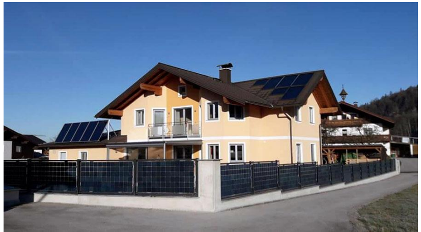
Figure 23 - Next2Sun GmbH. (2024). Solar fence in Adnet [Photograph]. Next2Sun. https://next2sun.com/en/solar-fence/
