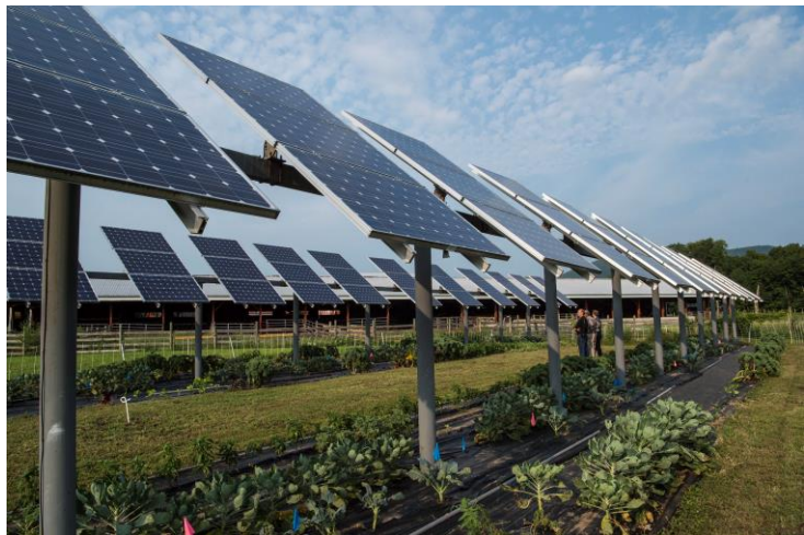
Figure 24 - Hyperion Systems LLC. (2025). UMass Amherst – Broccoli, bell peppers, kale, and Swiss chard growing under the dual-use solar array [Photograph]. Hyperion Systems LLC. https://hyperionsystemsllc.com/projects/umass-amherst/
