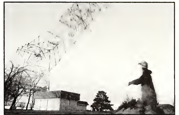
G ary Harmon, of Nationwide Towers in Henderson, Ky., walks away from the falling microwave tower Jan. 28 at the American Institute of Baking. The tower was removed because of liability and maintenance costs, and would be sold for scrap metal. (Photo by Clif Palmberg)
