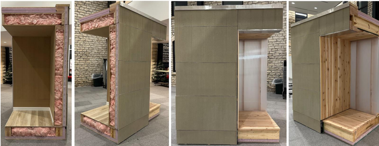
Figure 28. Completed Building Section Part 2
