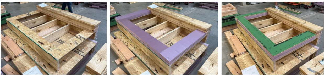
Figure 23. Installing Roof Rigid Insulation and ZIP Sheathing
