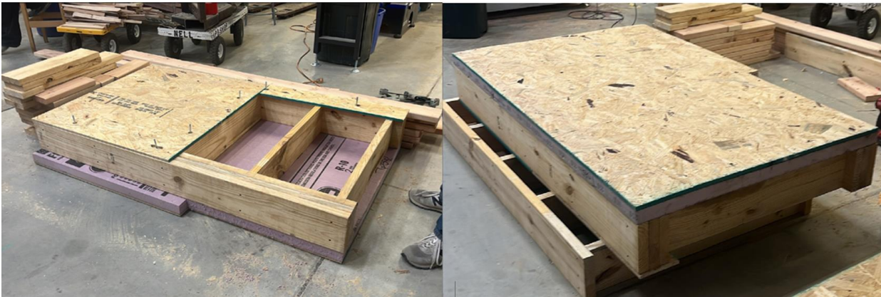
Figure 18. Floor Constructing Process Part 1
