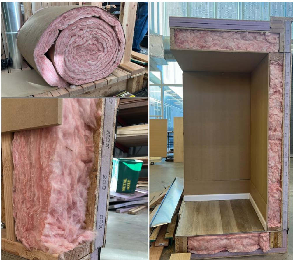
Figure 21. 5-1/2" Fiberglass Insulation
