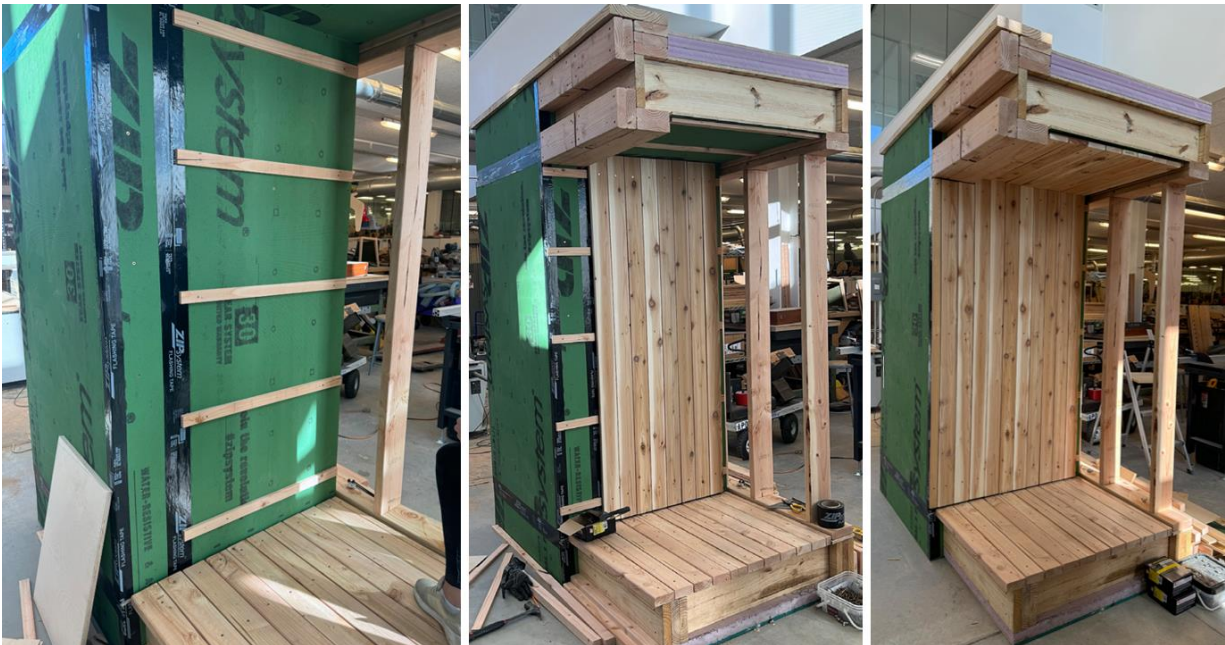
Figure 24. Implementation of Wood Cladding
