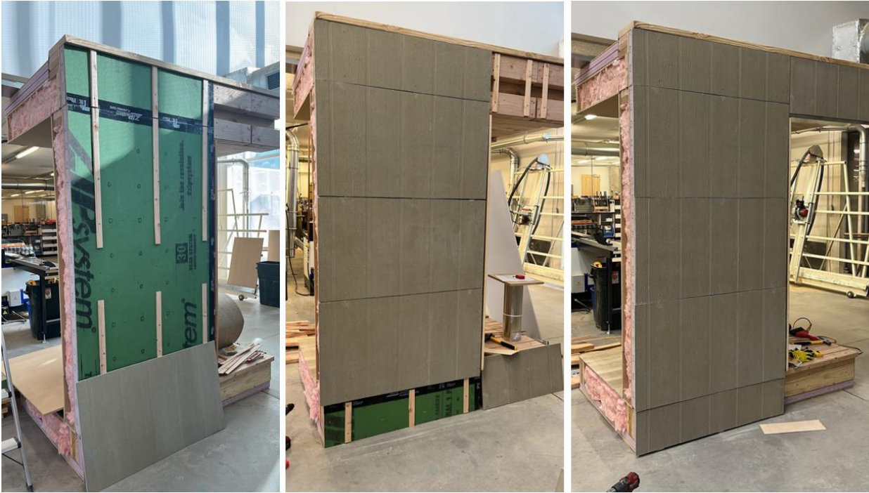
Figure 25. Implementation of Fiber Cement Cladding
