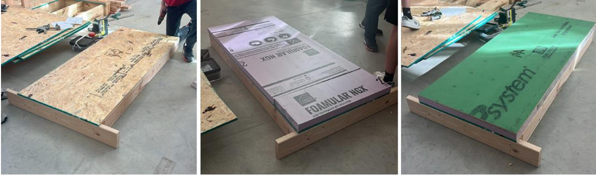
Figure 22. Installing Wall Rigid Insulation and ZIP Sheathing
