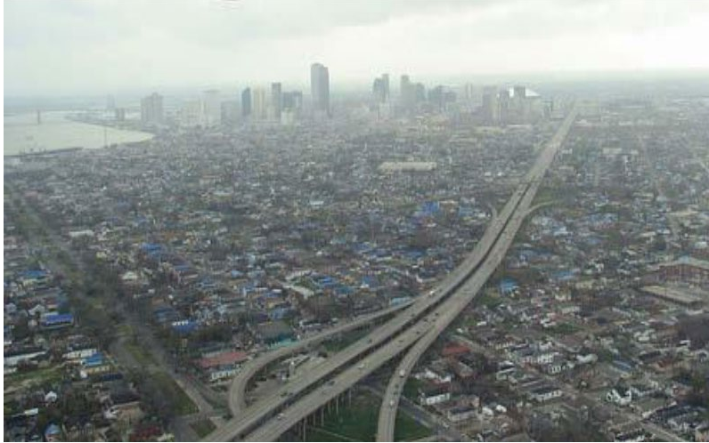
Figure 38. The I-10 Claiborne Highway, under the Claiborne Avenue expressway. Source Congress for New Urbanism (CNU) Highways to Boulevards Campaign, New Orleans
