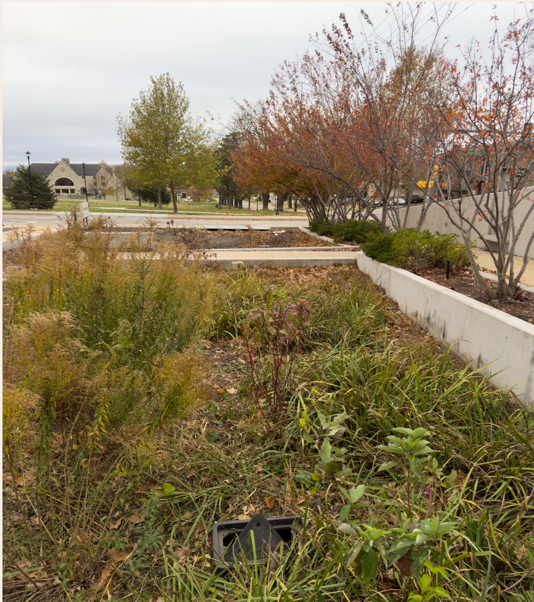
Fig 4.1 Engineering Bio-Retention Area after a storm (Freelove 2024).
