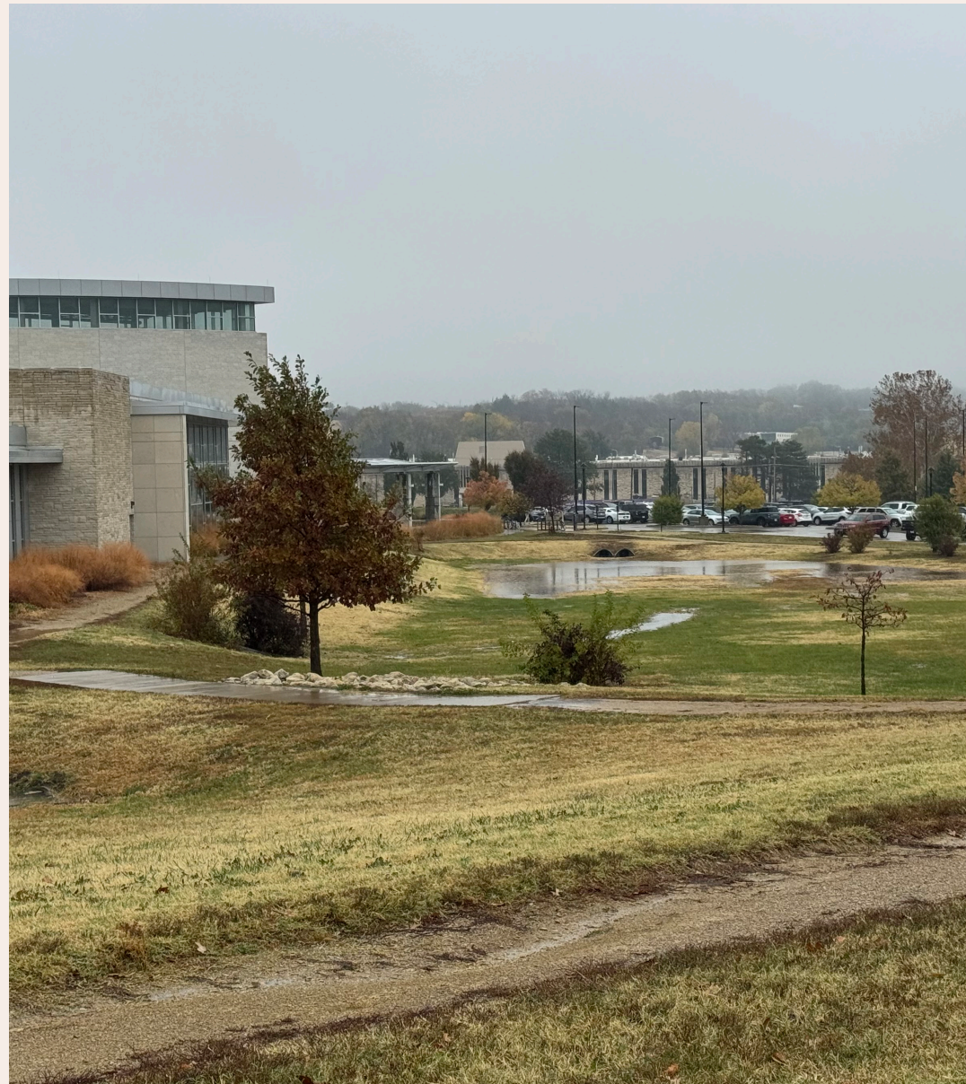
Fig 2.1 Peters Recreation Center's retention basin fills with stormwater runoff from the surrounding context (Freelove 2024).
