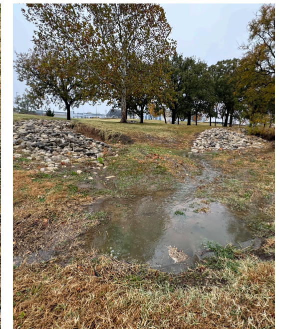
Fig 5.10 The swales on the west side of the Peter's Recreation site see large volumes of water moving through them (Freelove 2024).
