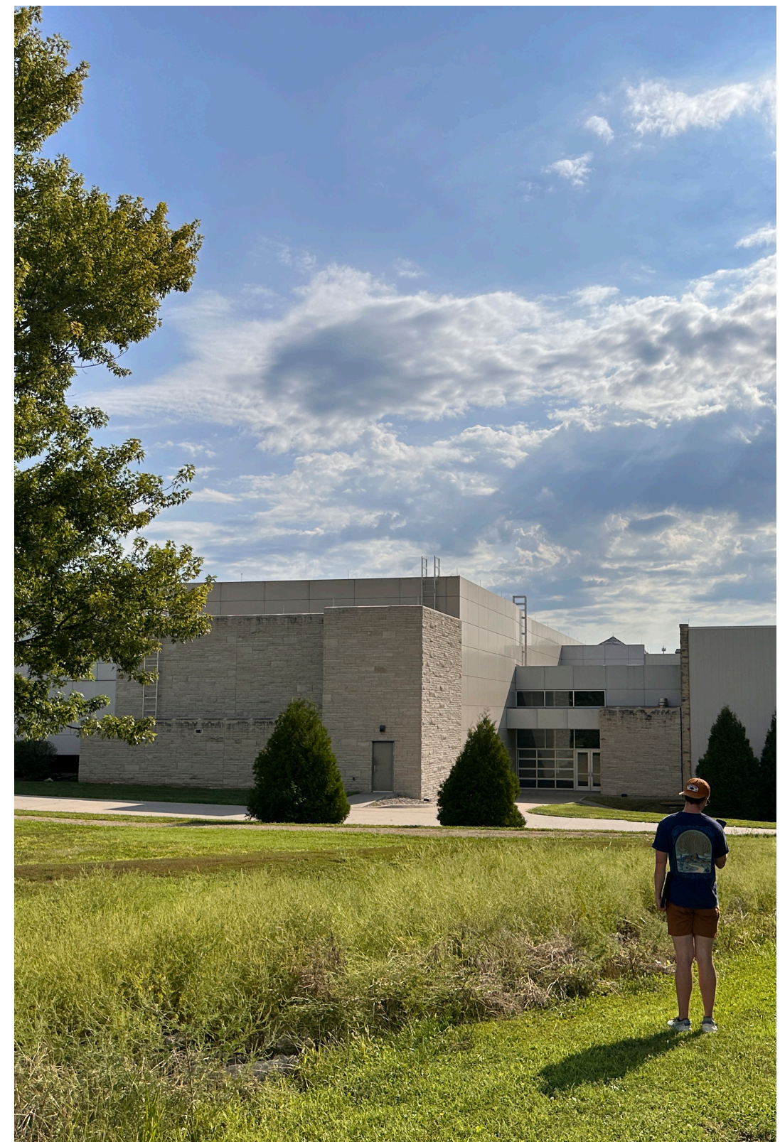
Fig 5.16 The swales provided great maintenance issues with many invasive species, and difficulty in maintaining the swale edges (Tilley 2024).
