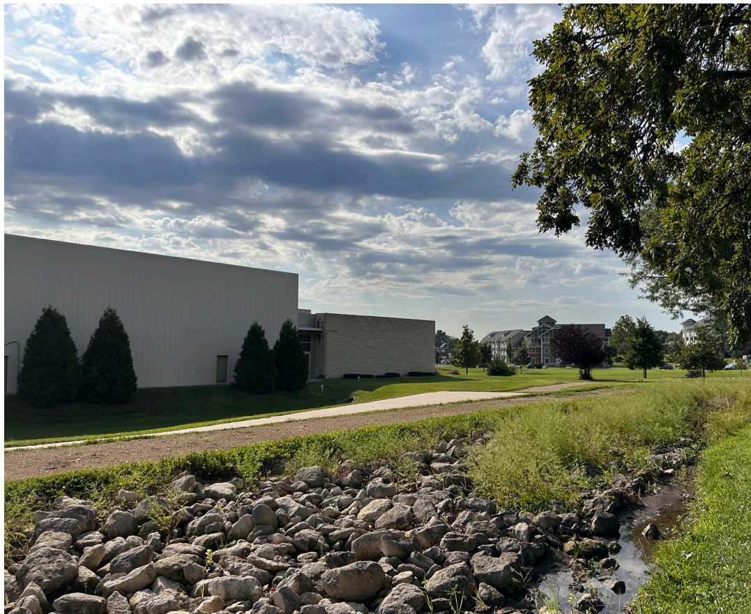
Fig 5.2 The swales around Peter's Recreation Center suffer from fast moving stormwater, leading to erosion and the addition of rip rap (Freelove 2024).
