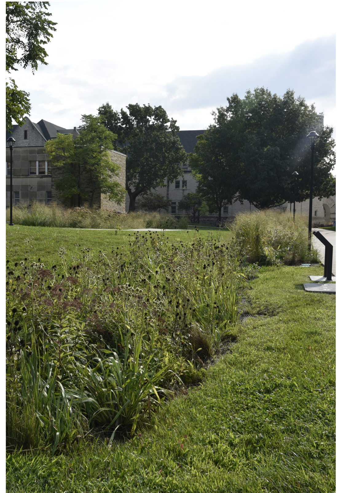
Fig 3.26 The Seaton Hall Bioswale is an example of GI that can take less time to manage than mowing due to its biodiversity and plant spacing (Goold 2024).
