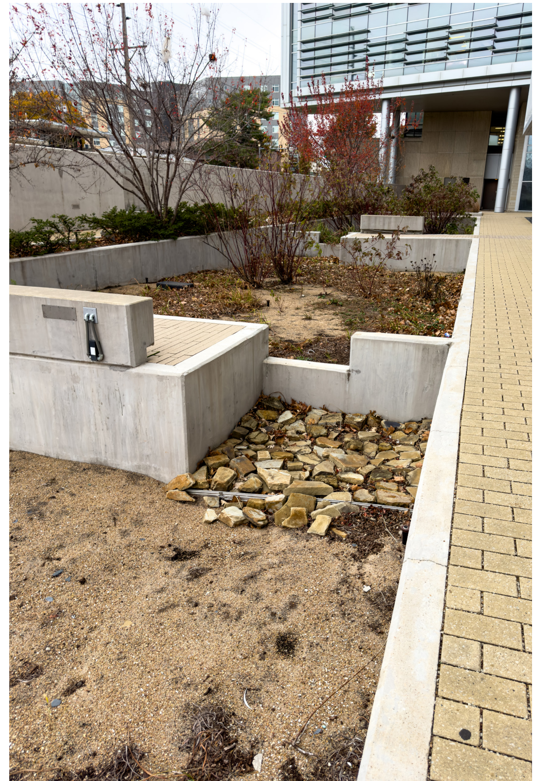
Fig 3.23 Eroded rock transitions between Engineering Bio-Retention Cells (Freelove 2024).
