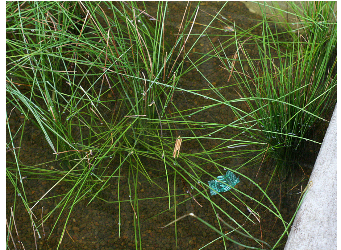
Fig 1.2 Rain garden fills due to large storm event, allowing for stormwater to infiltrate ("Bioswale" 2008).
