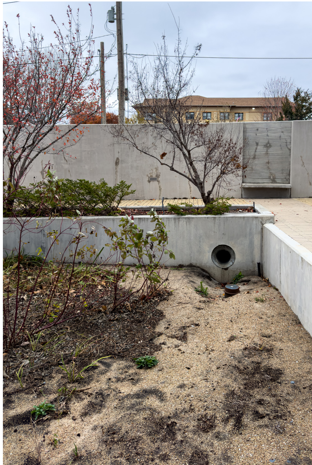
Fig 3.12 Engineering Bio-Retention Area (Freelove 2024).
