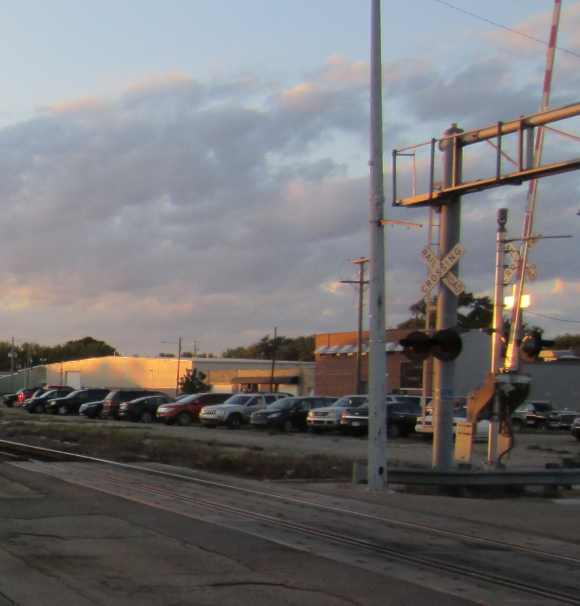
Figure 2.0.1 - View looking west at the N Kansas Avenue Railroad Crossing (Johnson, 2018)
