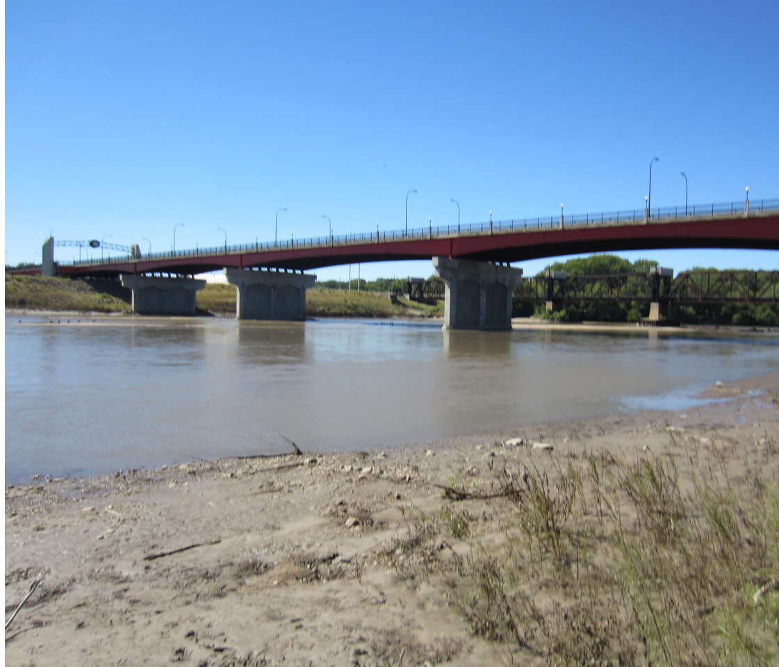
Figure 1.1.1 - Topeka Blvd. Bridge above the Kansas River (Johnson, 2018)
