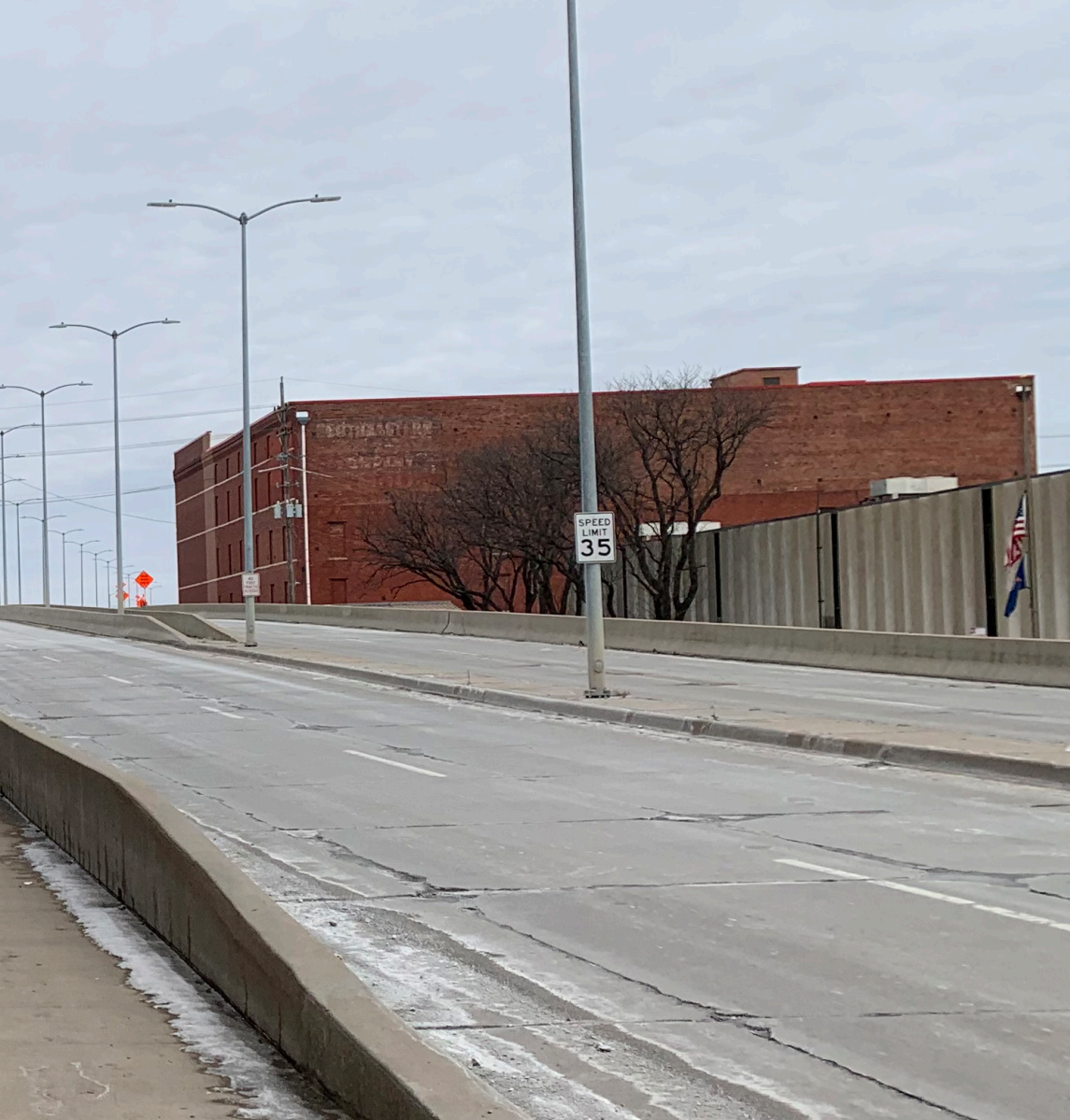
Figure 6.0.1 - View looking North at the Kansas Avenue Bridge South Landing (Johnson, 2019)
