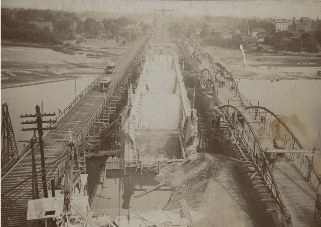
(Opposite) Figure 2.1.2 - Kansas Avenue Bridge, Topeka, Kansas (Kansas Historical Society, 1870's-1890's)
