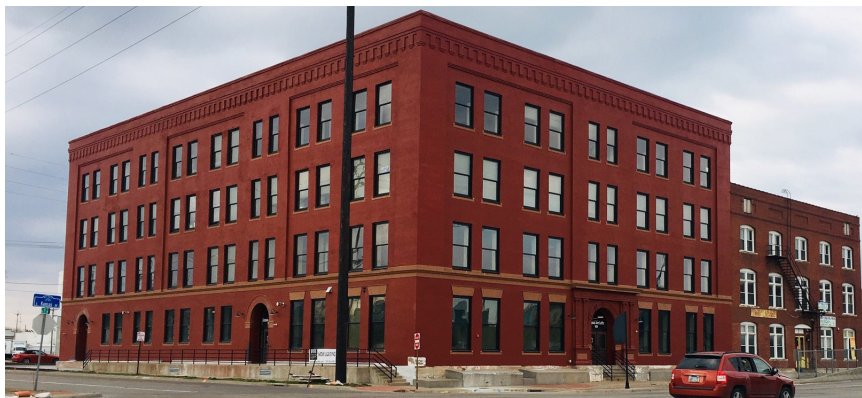
Figure 4.7.2 - Attractive Building Facade (Johnson, 2019)
