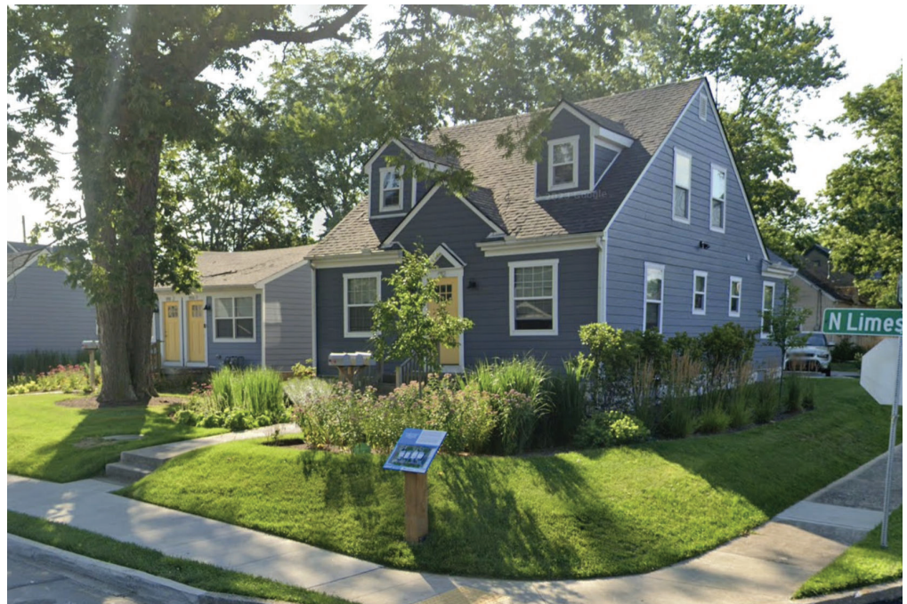
Figure 4.17 View of one of the stormwater management interventions in the Rain Gardens at 900 development
