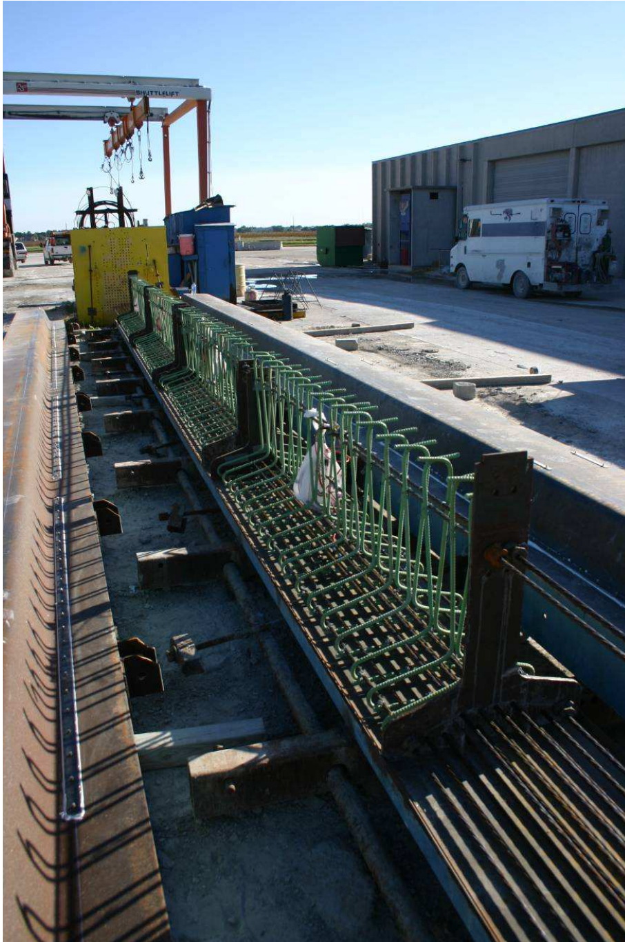
Figure 3.2 Tensioned beams' forms
