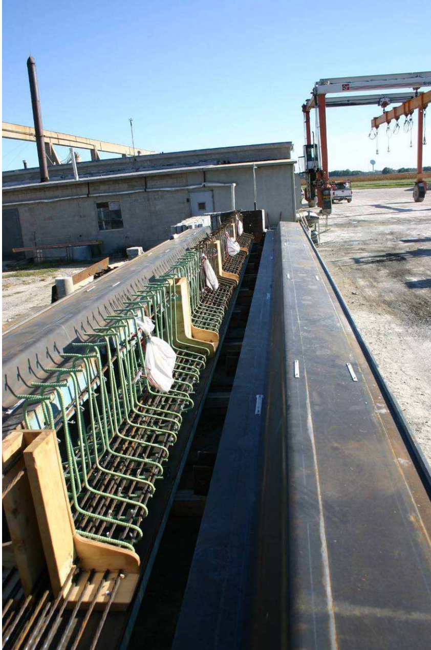
Figure 3.3 Untensioned beams' forms
