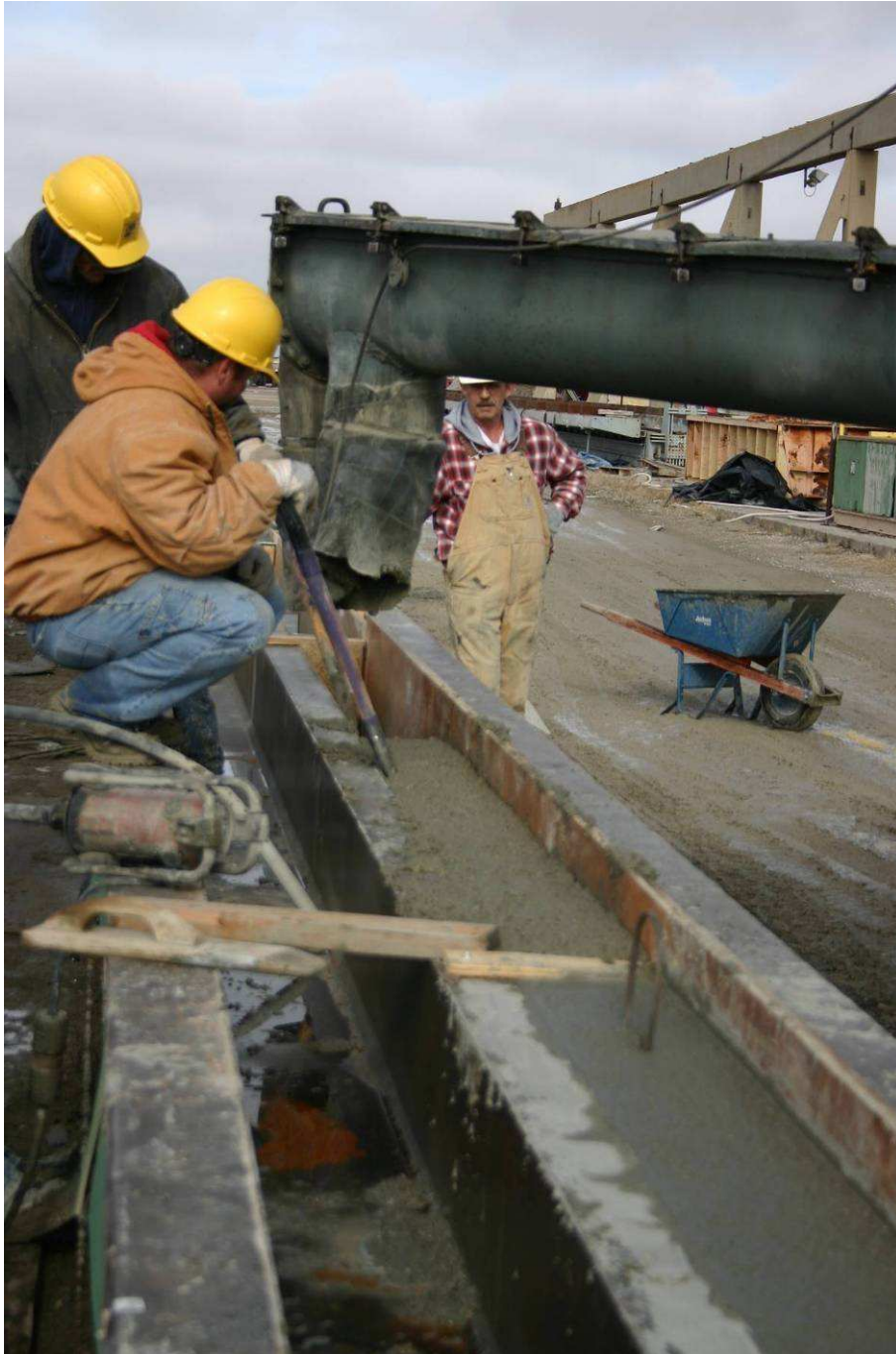
Figure 7.8 Casting of rectangular beam
