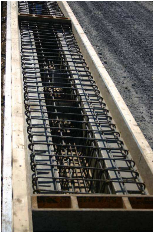
Figure 7.4 T-beams' form with reinforcement
