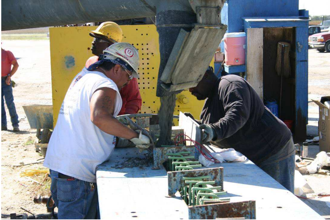
Figure 3.4 SCC beam being poured
