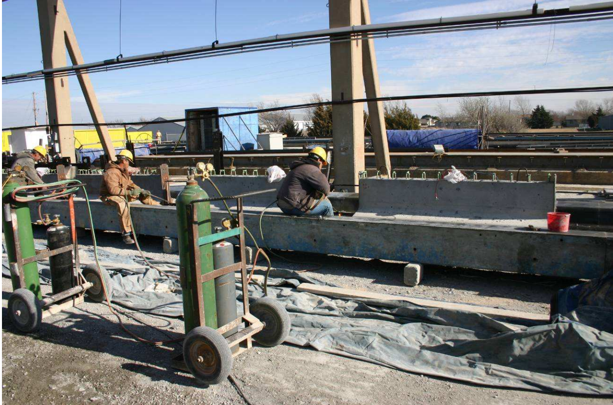
Figure 3.11 Workers simultaneously flame-cutting the prestress strand
