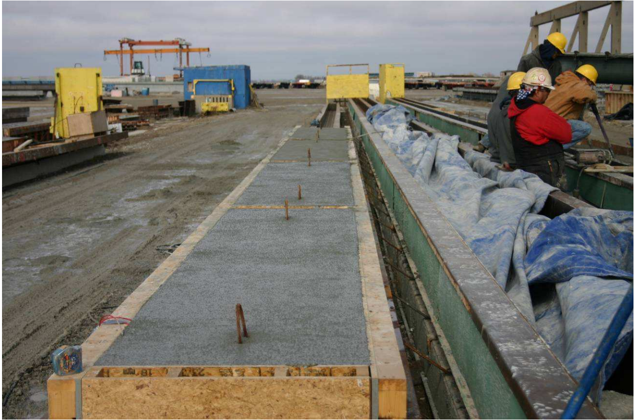
Figure 7.9 Finished T-beam specimens
