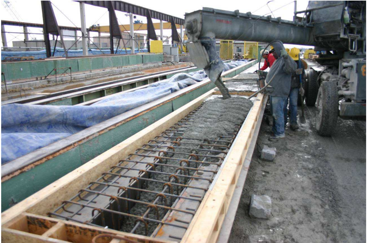
Figure 7.6 Casting of the T-beam specimens
