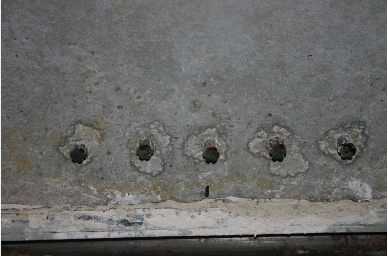
Figure 8.31 Discoloration of T-Beam ends
