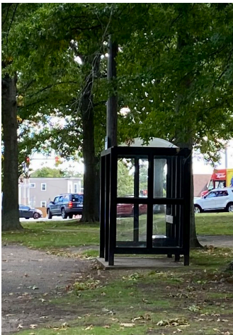
Fig. 6.13. Bus stop conditions at Peabody Circle.
