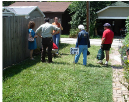
Fig 3.16: Gravel grass is a permeable paving type that allows for a flexible turfgrass lawn to be used as parking if needed. Photo by Marcus de la Fleur, used with permission.
