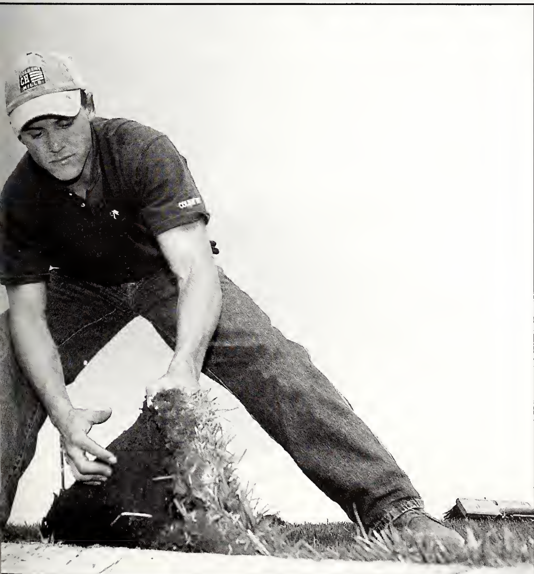
Packing a piece of fresh sod next to the cart path, Green lays the sod by hand to ensure it is flush to the path's edge. (Photo by Evan Semon)
