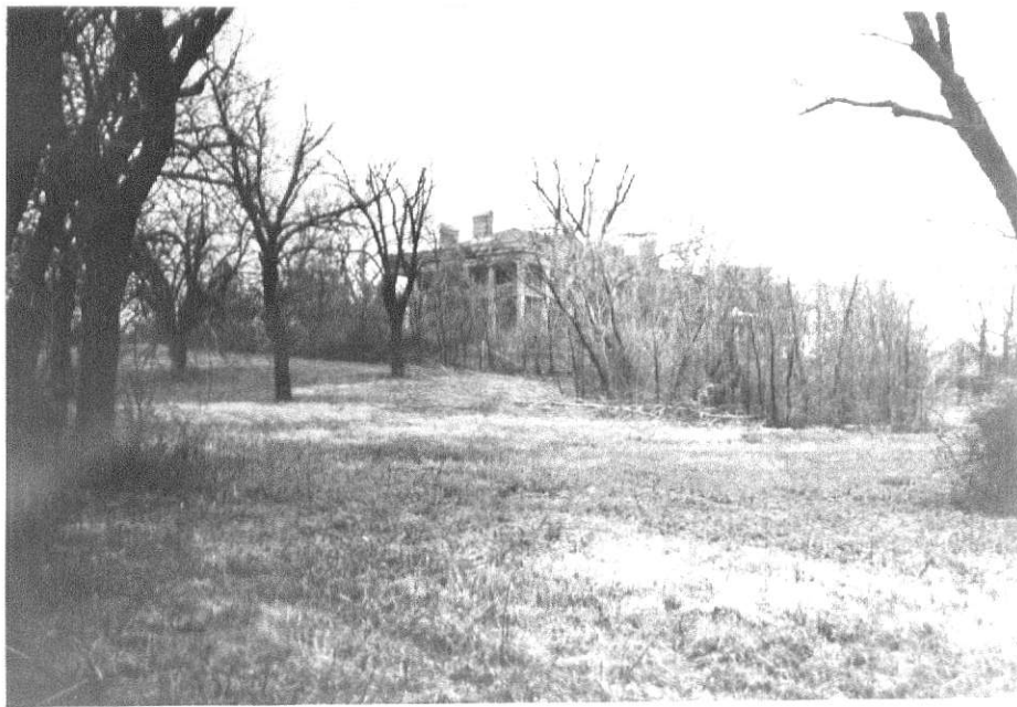
Figure 21. The Mansion as Seen from the Southwest Corner of the Site.
