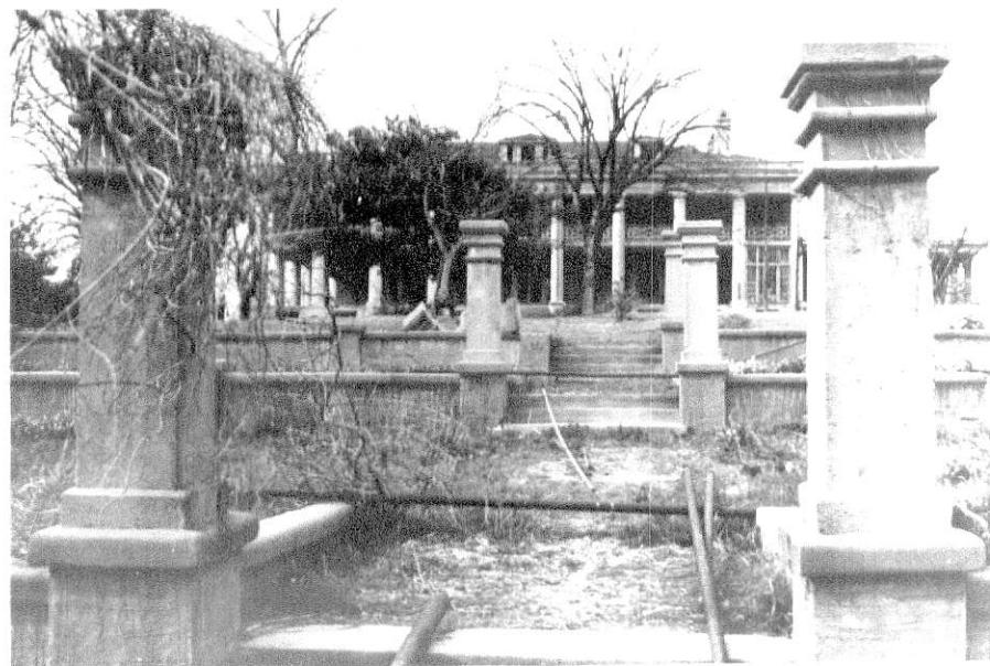
Figure 18. The Sight Line of the Formal Planting Terraces Ends Aimlessly on One of the Columns of the Mansion. The Music Room Doorway at the Mansion is visible at the left.
