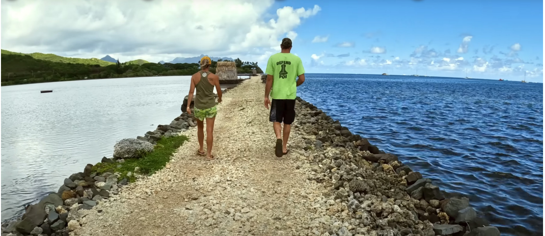
Fig. 5.9 Fishpond system The Hawaiians developed advanced aquaculture systems through a series of manmade ponds that ranged in salinity. Loko Kuapa consisted of a sea wall with an opening covered by a woven grate.
