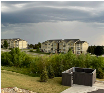
Figure 6.9. View of Drainageway
