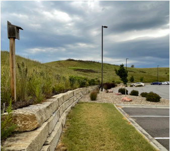
Figure 6.17. Retaining Wall around Parking Lot
