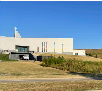
Figure 6.8. FCC Loading Area
