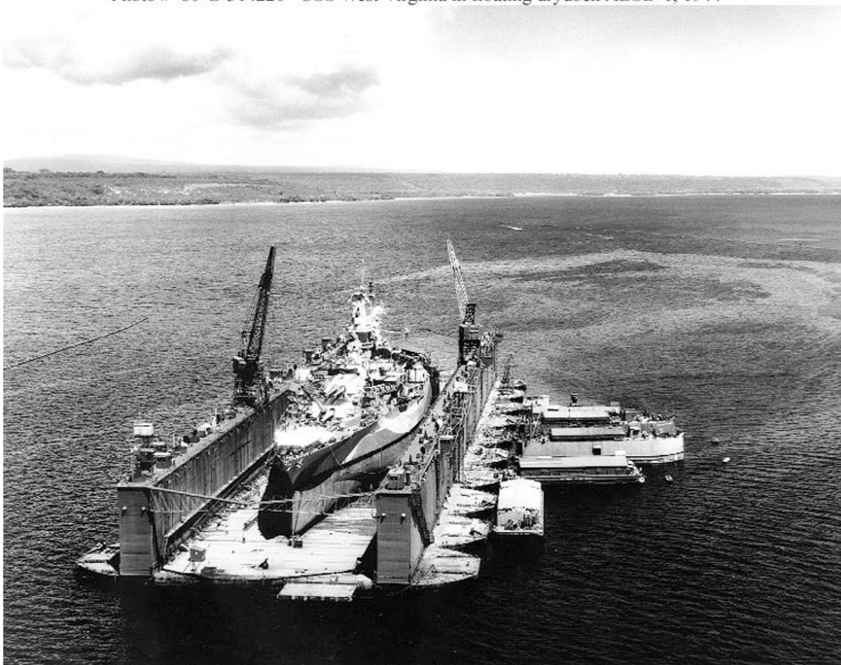
Figure 3. ABSD-1 with *West Virginia* docked off Espiritu Santo in the New Hebrides Islands. This dry dock is of the open-ended design where the ship sails into the dock when it is underwater and then is raised by pumping mechanisms. Photo 2 at the end of the chapter shows YFD-2 *New Orleans* which is of the gated design which involves flooding of the compartment itself and then pumping the water out. (Courtesy of the Naval Historical Center)
