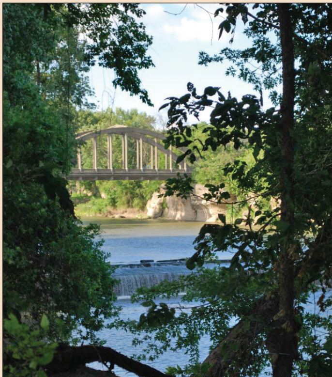
Bridge over the Neosho River in Humboldt.
