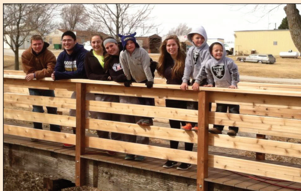
Randolph's bridge project funded through a Get It Do It Grant.
