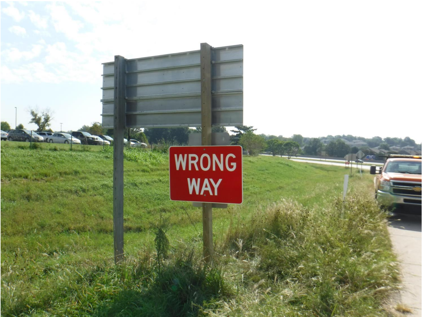
Figure C. 31: Installation of 1st Oversized and Lowered Wrong Way Signs on Wanamaker Rd North Ramp
