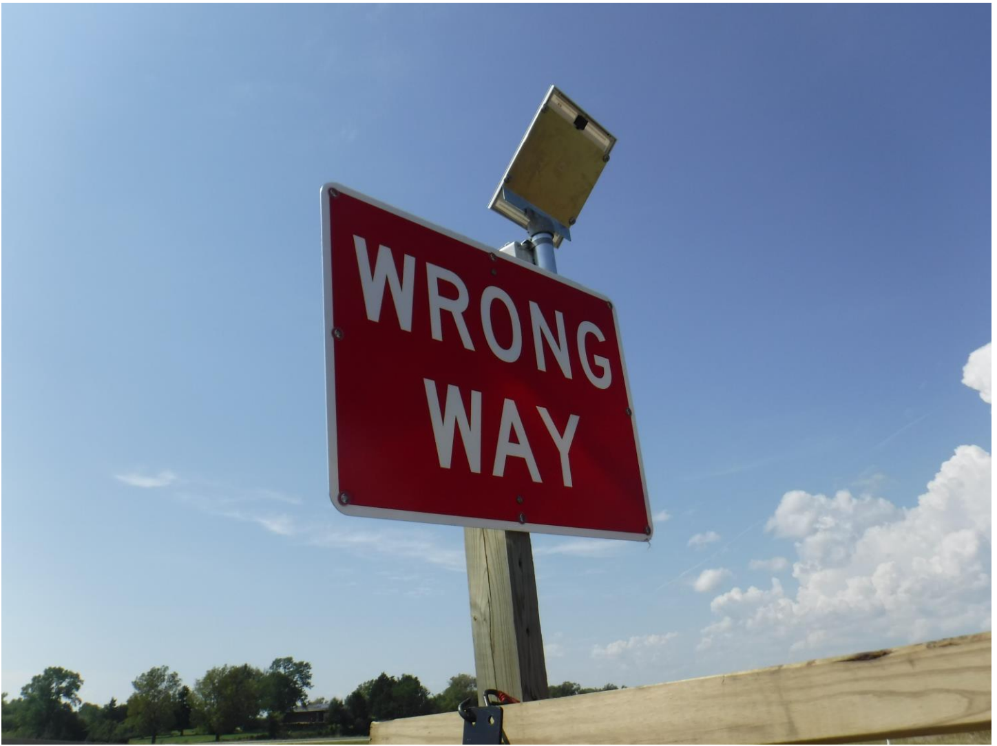
Figure C. 34: Installation of Flashing LED Wrong Way Sign at Auburn Rd Ramp
