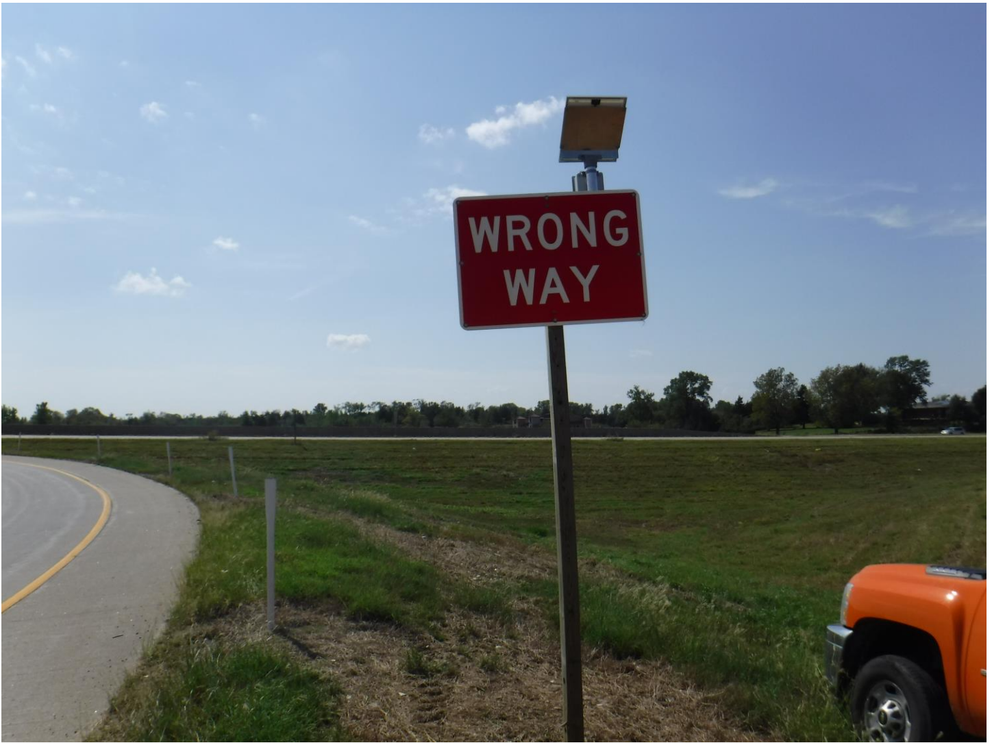
Figure C. 35: Installation of Flashing LED Wrong Way Sign at Auburn Rd Ramp
