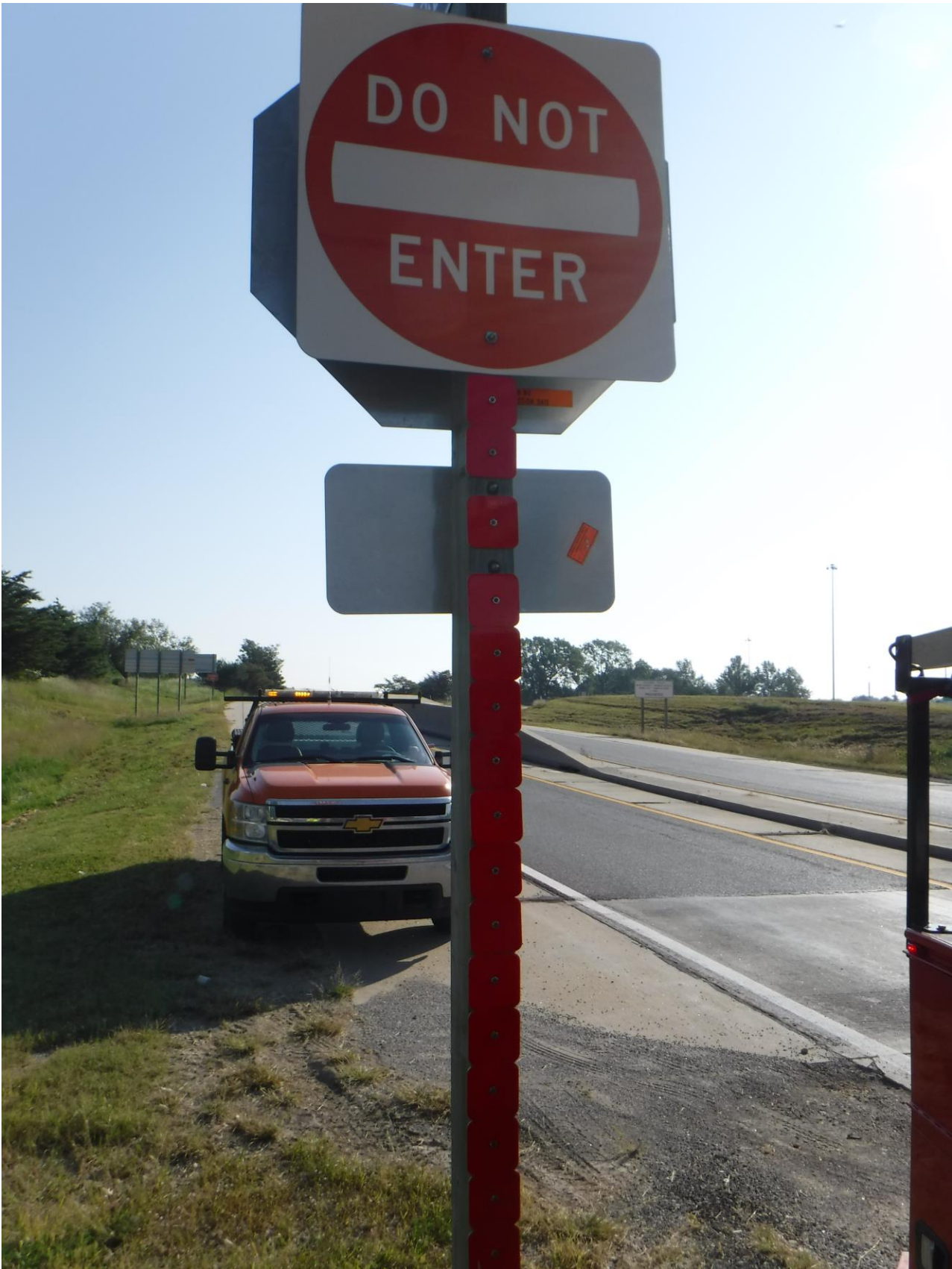
Figure C. 29: Installation of RRFDs on Gage Blvd
