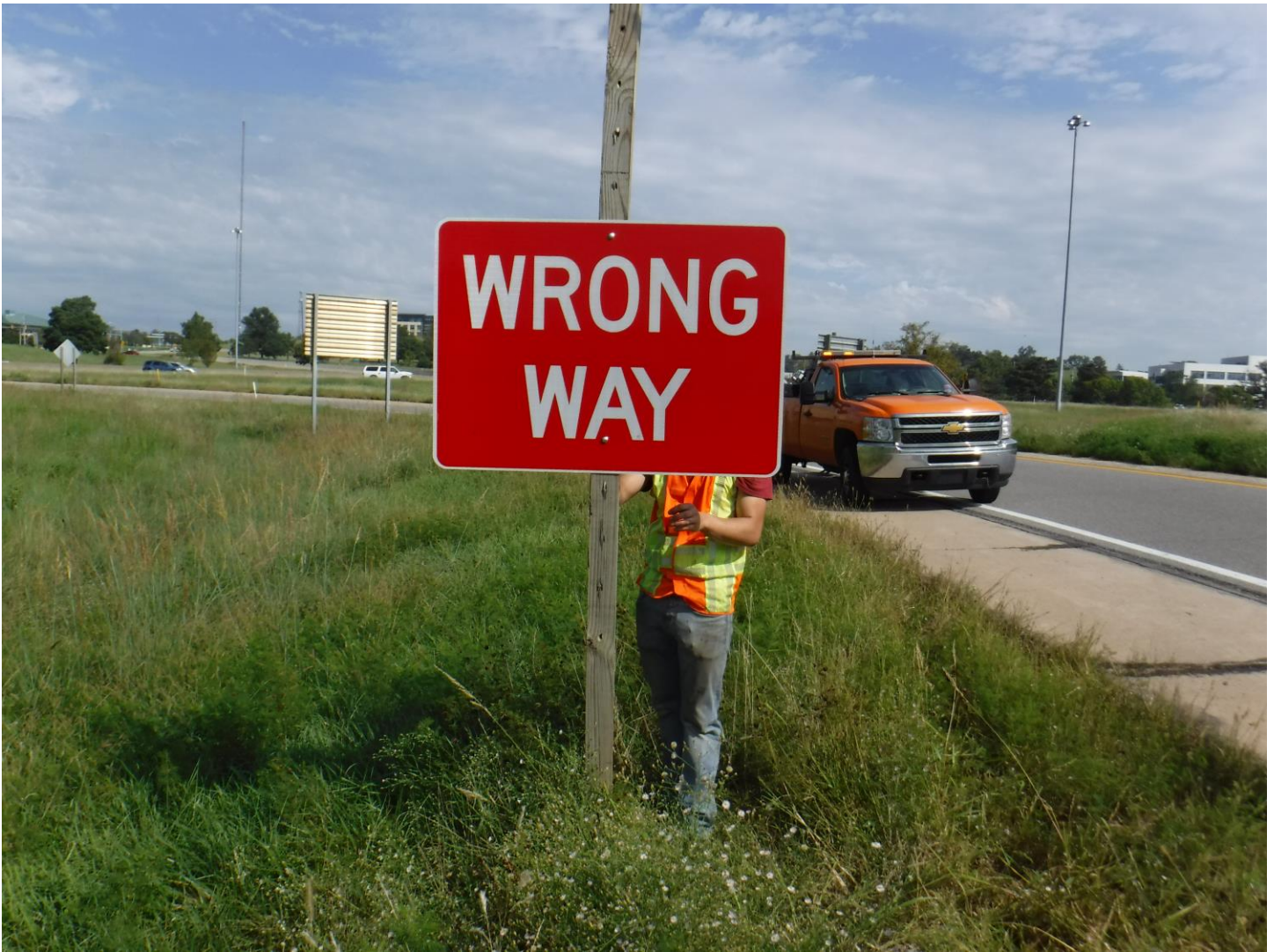
Figure C. 33: Installation of 2nd Oversized and Lowered Wrong Way Sign on Wanamaker South Ramp
