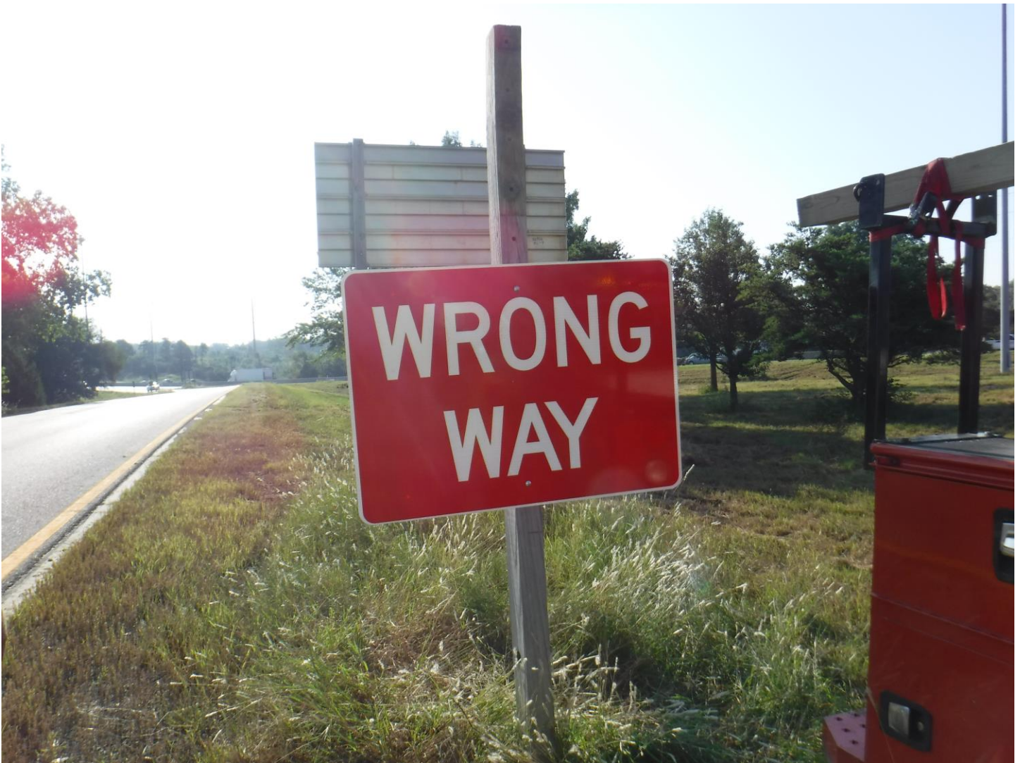
Figure C. 28: Installation of Oversized and Lowered Wrong Way Sign at Gage Blvd Ramp
