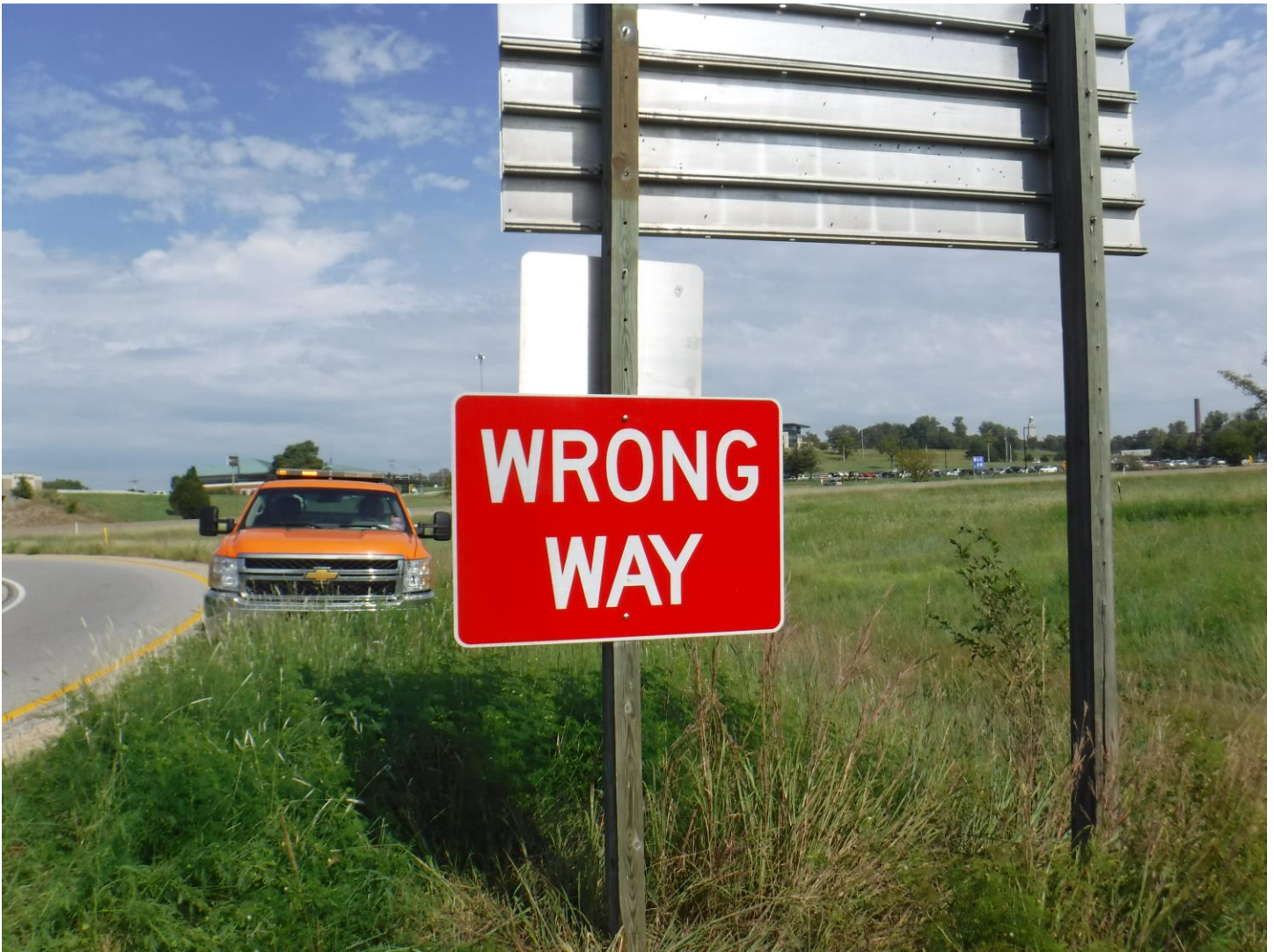
Figure C. 32: Installation of 1st Oversized and Lowered Sign at Wanamaker Rd South ramp
