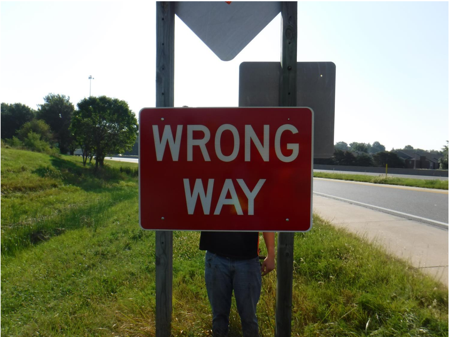
Figure C. 30: Installation of 2nd Oversized and Lowered Wrong Way Sign on Wanamaker Rd North
